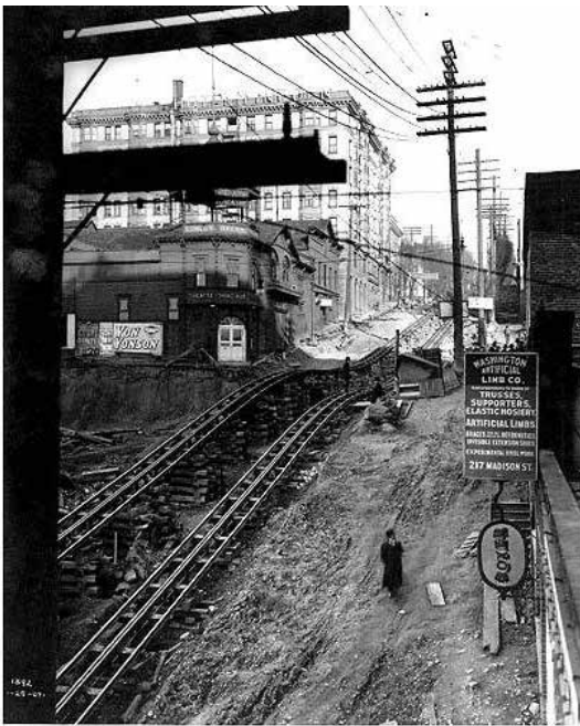
Madison Under Construction
