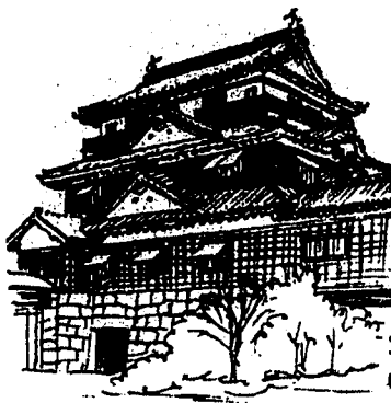
Figure 2-40. Matsuyama Castle, rebuilt in 1854.
