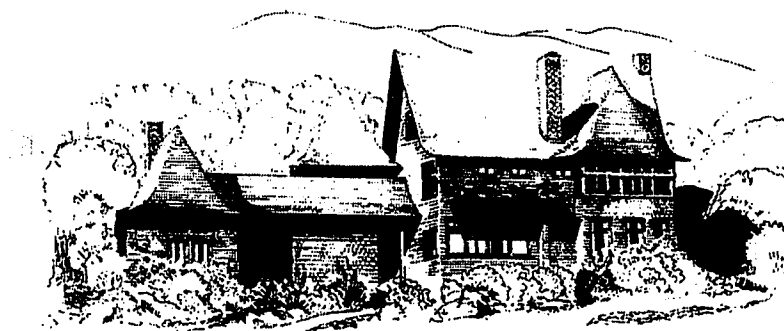
Figure 2-15. Bernard Maybeck, the Keeler house, Berkeley, California, 1894.
