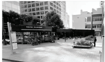
5 1111 3rd Ave 3rd & Spring 1111 3rd Ave Plaza, Shopping Arcade, Arcade
