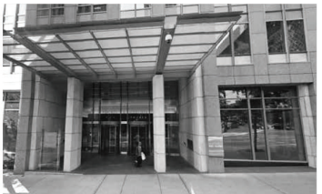
10 Fourth & Madison Building 4th & Madison 925 4th Ave Public Atrium, Hillclimb Assist
