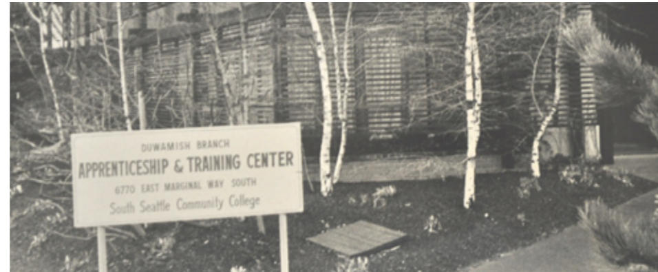
Fig 4.10 Duwamish Apprenticeship Center in Seattle's Georgetown neighborhood from 1969
