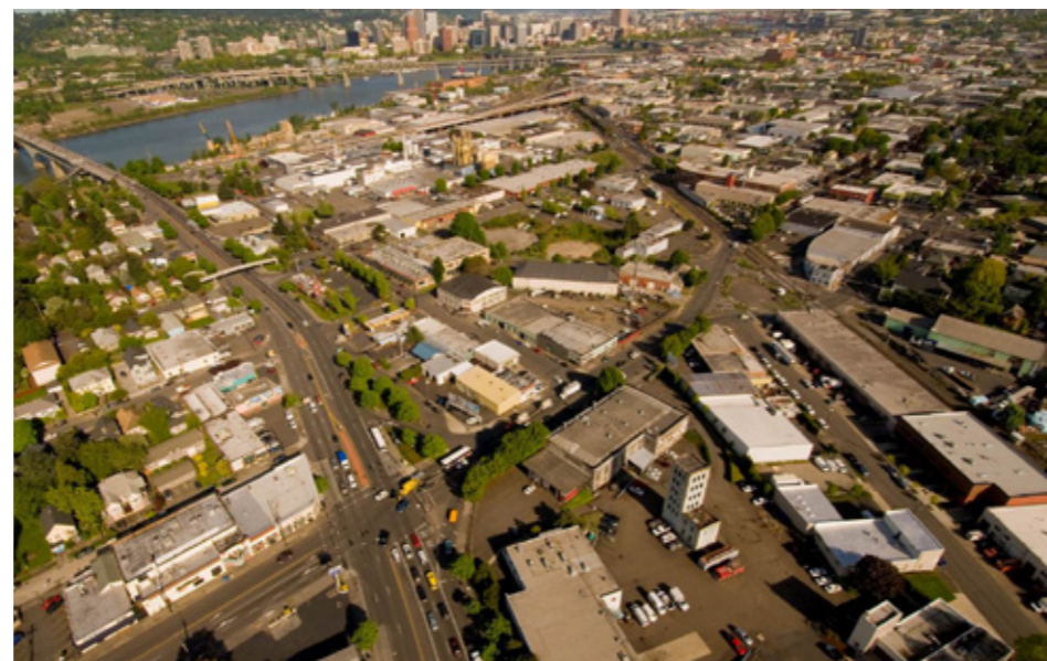
Fig 2.8 Aerial view of the Central Eastside District
