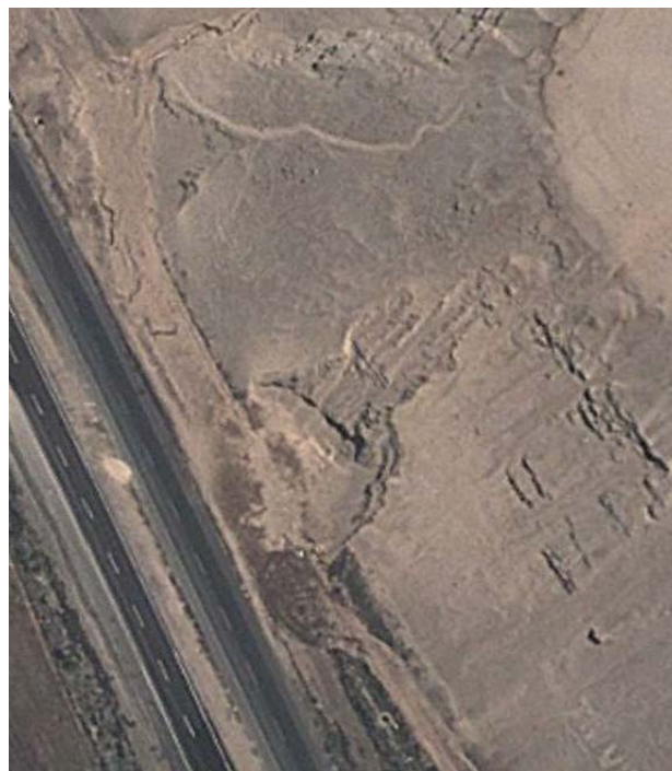
Figure 4. Debris/earth avalanche, Coastal Plains. Image from Google Earth.
