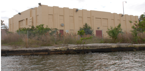
VACANT BUILDING: owned by Department of Parks and Recreation
