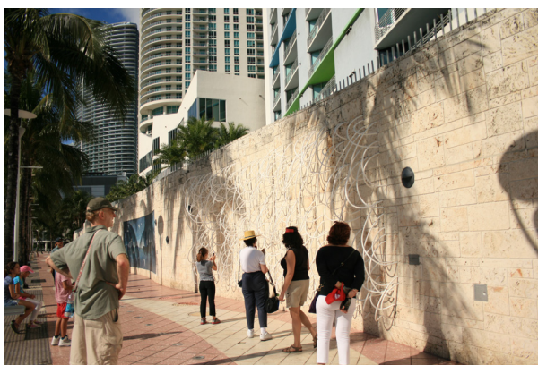
FIGURE 18: City of Miami Riverwalk, portion built to date, Lower River Zone
