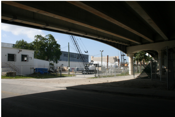
FIGURE 44: Existing 12th Ave. Bridge, under utilized space for pedestrian enhancements.
