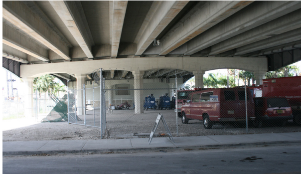
EXISTING 12TH AVE BRIDGE
