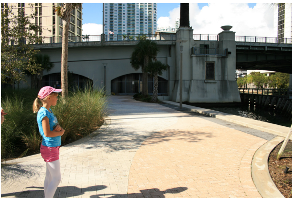
FIGURE 21: Built City of Miami Riverwalk segments that currently are not using bridge underspaces.
