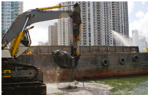
FIGURE 24: Images of the dredging process.
