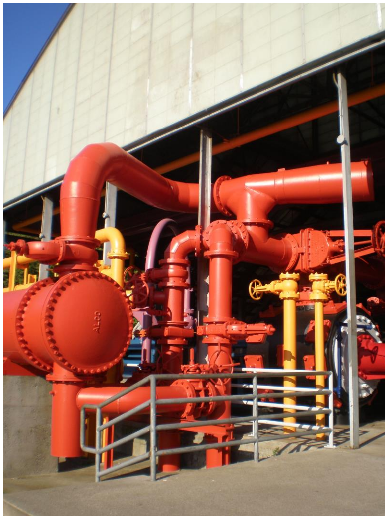
Fig. 6.4 Gas Works Pump House, wiki commons
