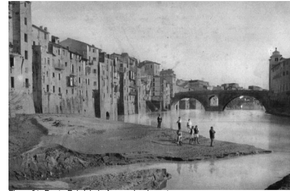
Figure61: Ponte Fabricio before embankments.
