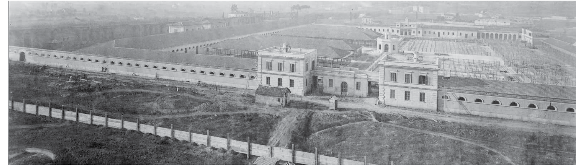
Figure90: Campo Boario under construction.
