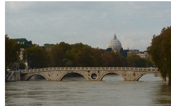
Figure158: Ponte Sisto during Tiber flooding of 2008.
