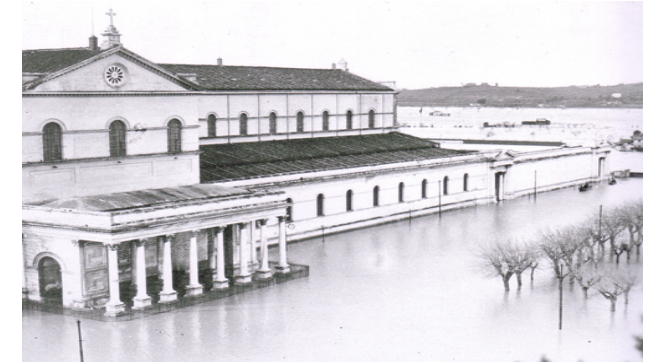
Figure31: Basilica di San Paolo flooded.
