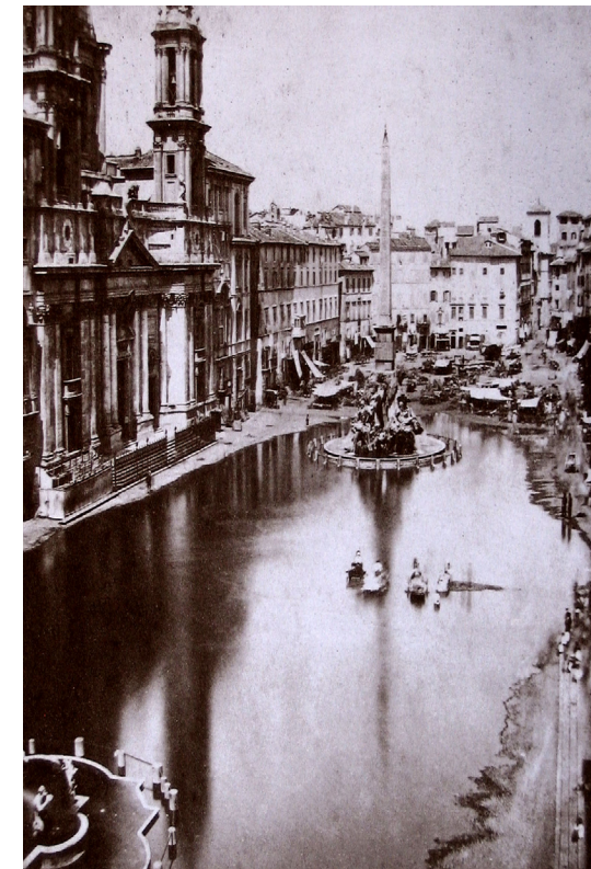
Figure30: Piazza Navona flooded.
