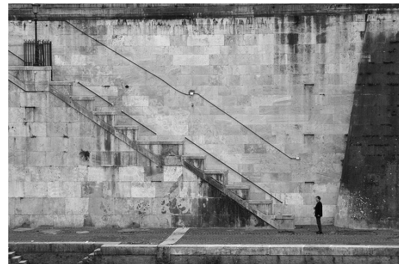
Figure60: Embankment access stairs and scale.
