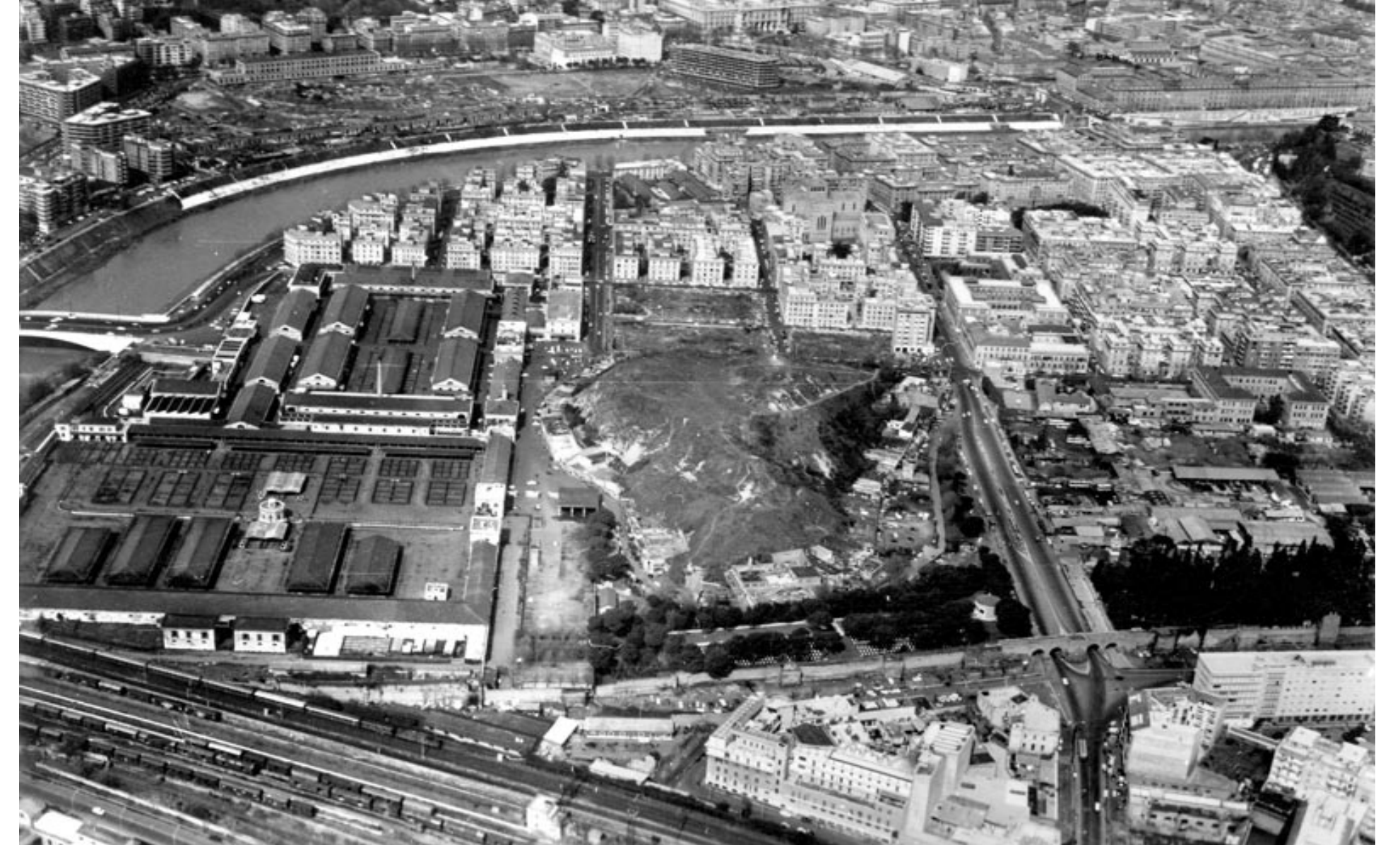
Figure78: Aerial view of Monte Testaccio and Mattatoio looking north.
