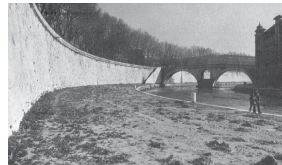
Figure62: Ponte Fabricio after embankments.
