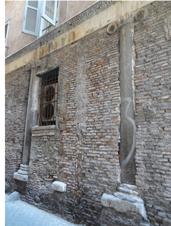
Figure212: Street wall along Via Capo di Ferro, showing the fluidity of the city fabric and the way a column can become a window frame.
