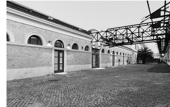
Figure103: View of architecture school Universita di Roma Tre, after redevelopment.
