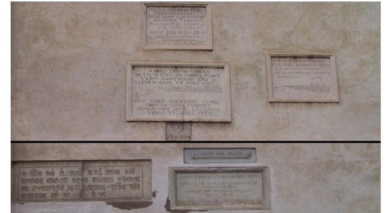
Figure38: Number 16: Church of S Maria Sopra Minerva flood markers.
