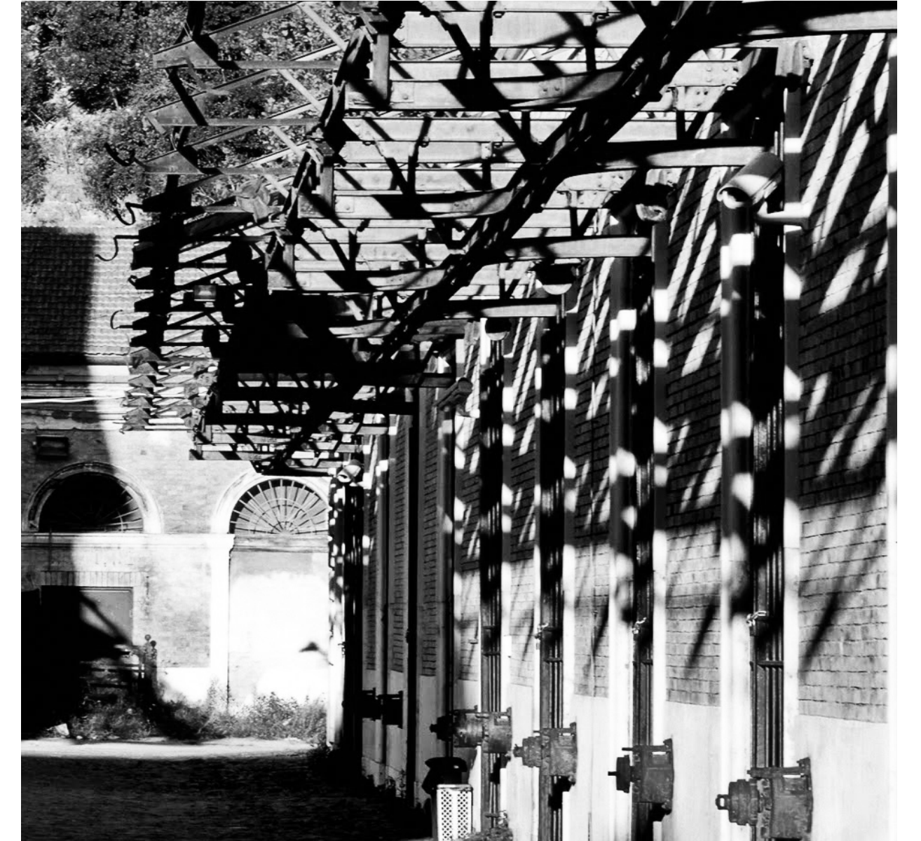
Figure106: Overhead rail system used to transport slaughtered livestock carcasses from one building to another in the Mattatoio.
