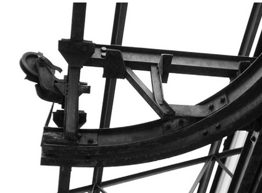
Figure99: Detail of the overhead rail system in the Mattatoio.
