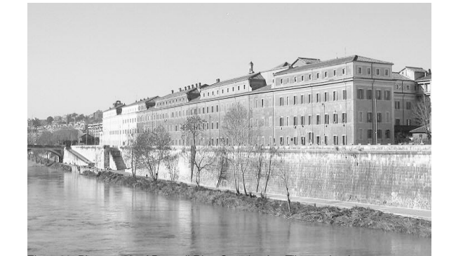
Figure20: Photograph of Porto di Ripa Grande after Tiber embankments.
