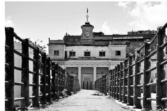
Figure89: Borsa Building in Campo Boario looking down the central axis.
