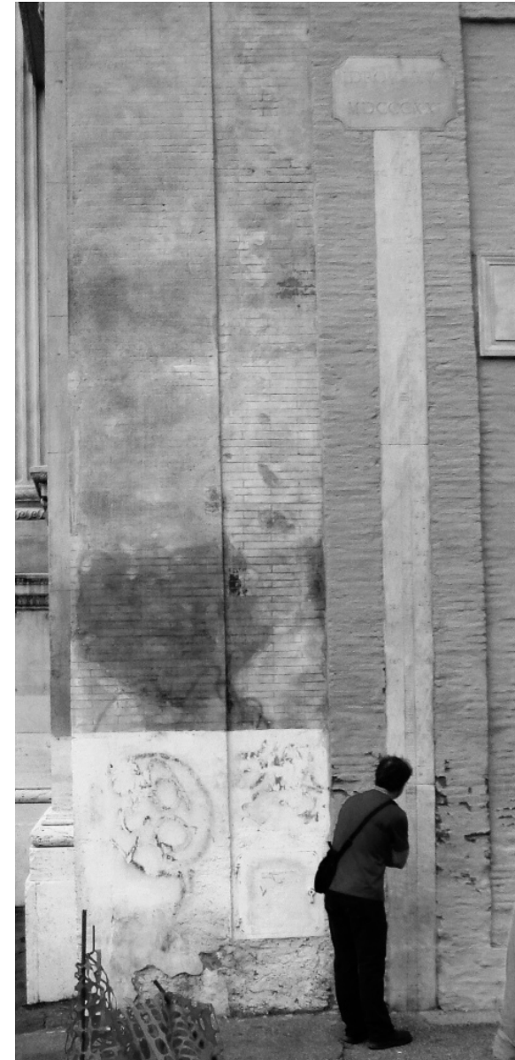
Figure34: Idrometro: On the facade of the Church of San Rocco Church [full view].
