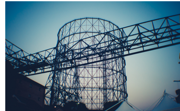
Figure201: Gasometro complex and its structural expression and relationships.
