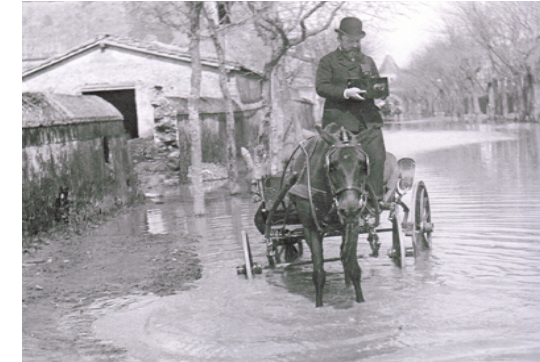
Figure29: Via Ostiense flooded.
