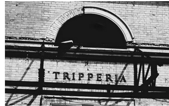
Figure93: Tripperia entrance door and overhead rail system in the Mattatoio (tripe).
