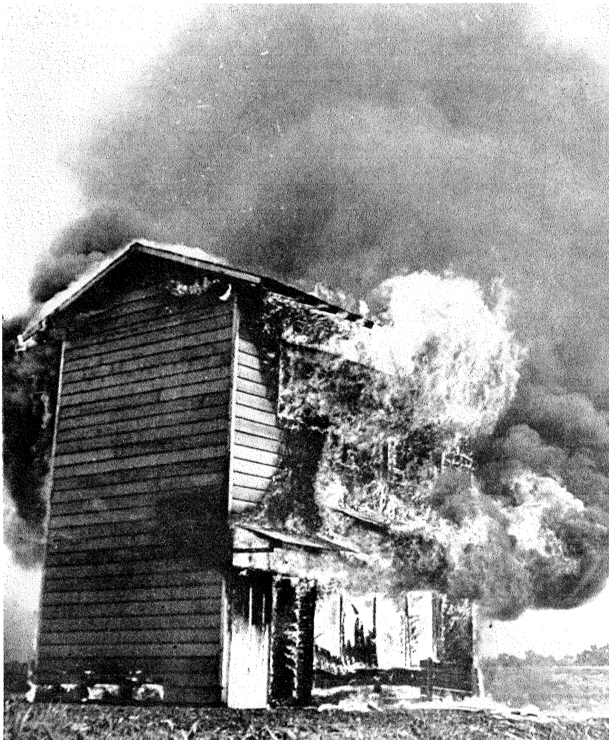
Photo 1: Dugway Proving Ground, Testing the M-69 incendiary bomb on a model enemy building.
