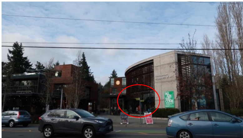
The floor-to-ceiling window is in the red circle, the photo is credited to the researcher.
