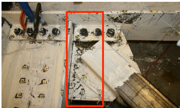
a. Complete Fracture of Beam to Gusset Plate Weld
