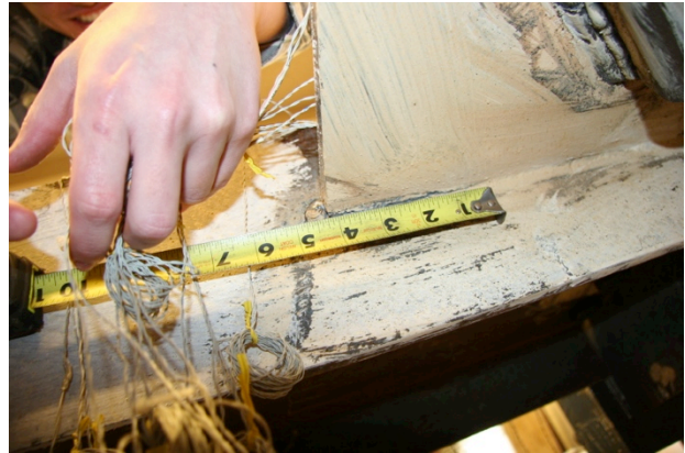
b. 4.125 in. (bottom) & 0.75 in. (top) weld crack at -1.3% drift
