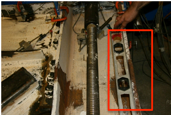
a. Local Buckling (B1) on West Flange
