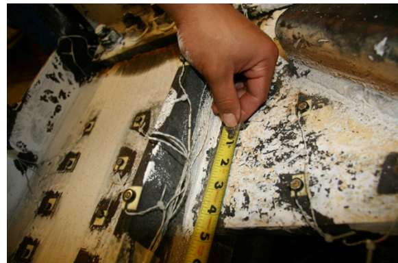
f. 4.25 in. weld crack (top) at -2.9% drift
