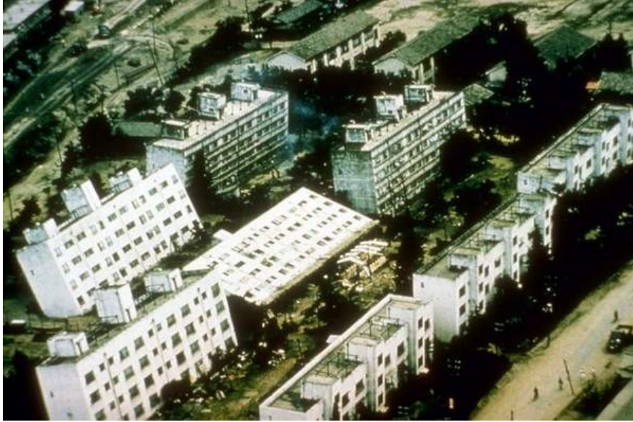
Figure 2.1: Collapse of tall buildings as a result of liquefaction-induced bearing failure during the 1964 Niigata Earthquake (USGS)
