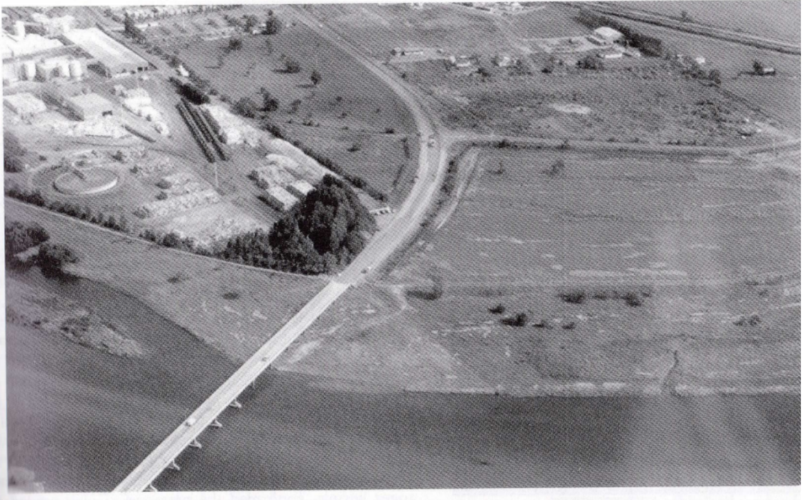
Figure 3.10: Aerial view of Landing Road Bridge site, looking northwest. Ground cracks near the bridge abutment, extending a 300m inland, are marked by lighter-colored sand ejecta. (Berrill et al., 2001)
