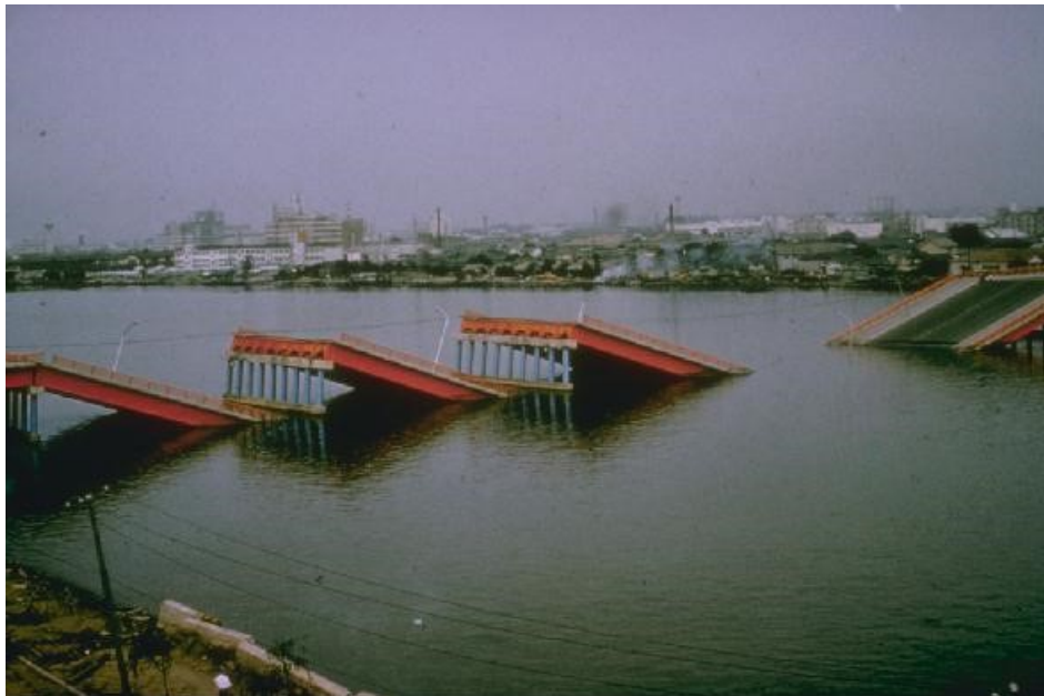
Figure 2.2: Collapse of the Showa Bridge, due to lateral spreading, during the 1964 Niigata Earthquake (USGS)
