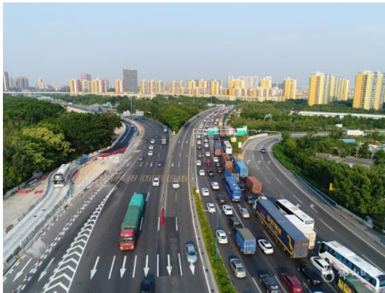
Figure 5.8 Directional Congestion on Guangfo Express Road 5
