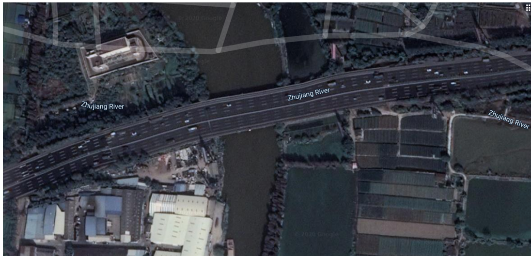
Figure 5.7 Satellite View of Guangfo Express Road
