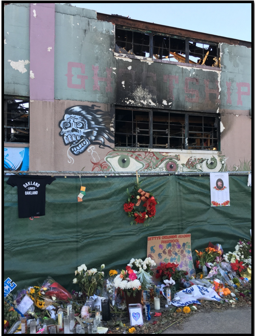
Figure 41: Memorial in front of Ghostship site. Photo by author, 2016.
