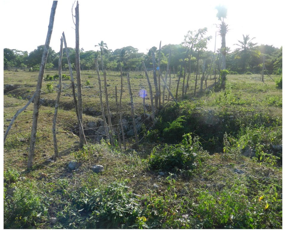
FIGURE 25: Foundation remnant; 12' x 12' hole
