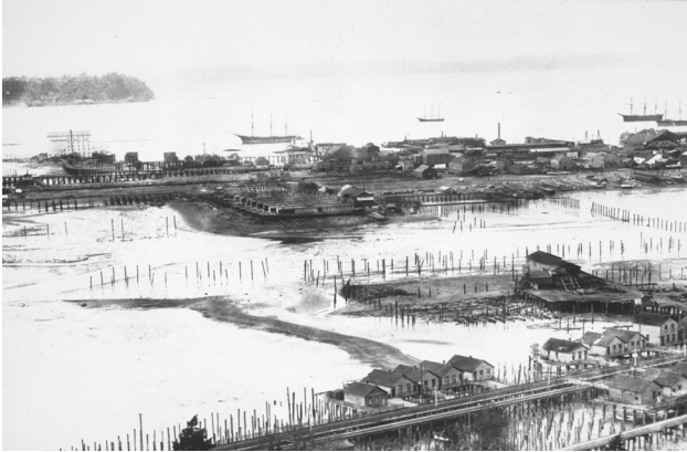
Figure 6.4 : Sodo Infill. Infill and construction of the SoDo industrial area over tidal flat and marsh area. [3]
