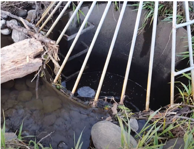
Figure 5.4 Licton Spring culvert
