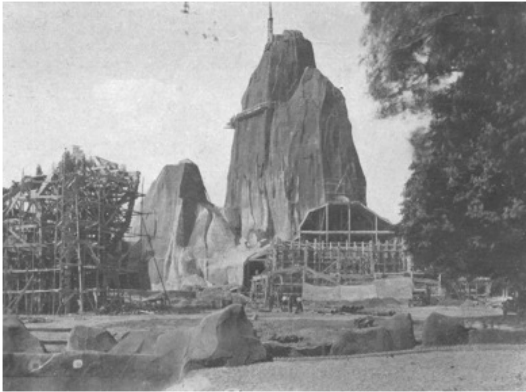
Figure 13: Construction of the “Big Rock”, Vincennes Zoo, 1934.
