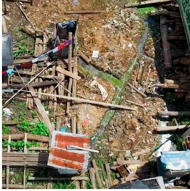
Figure - 31 - Low river season sewage swale
