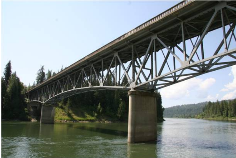
Figure 4.3: Photo of BR 31/36 over Metalin Falls River
