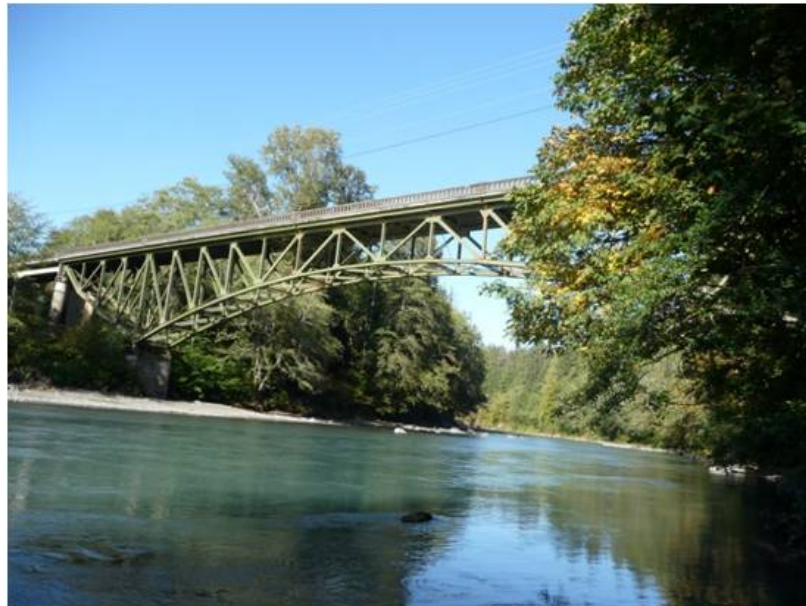
Figure 4.5: Photo of BR 101/217 over Hor River
