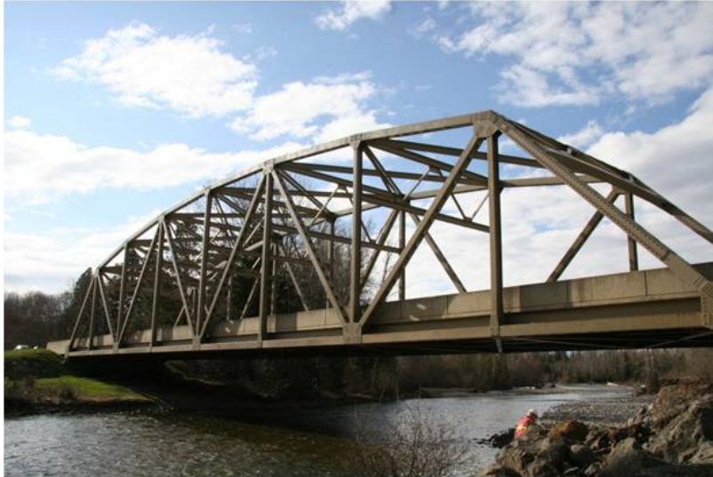
Figure 4.1: Photo of BR 90/134N over Cle Elum River
