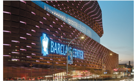
Figure 24 Barclays Center_Facade Panels
