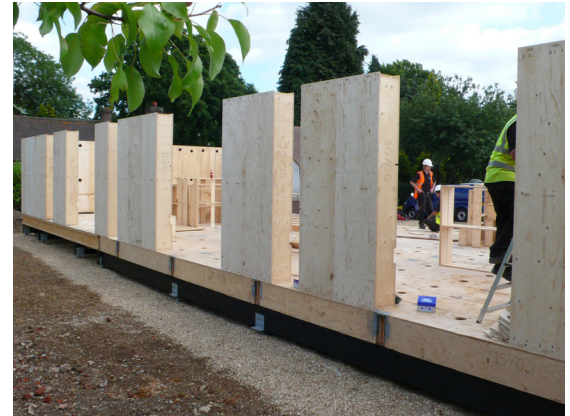
Figure 12 Cassettes Form Walls
