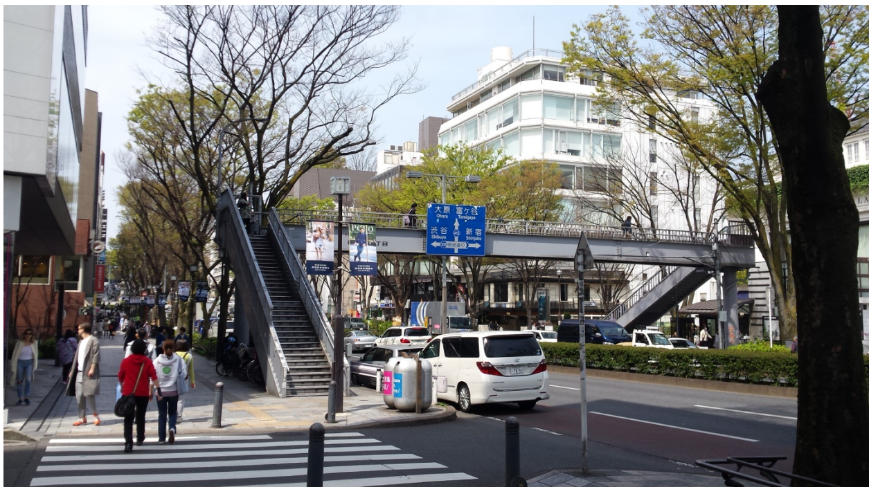
Figure 15: Pedestrian Flyovers became common features in post-war urban development.
