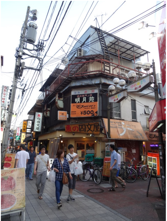
Figure 24: Building forms are highly individualized without reference to rigid planning or a unifying framework
