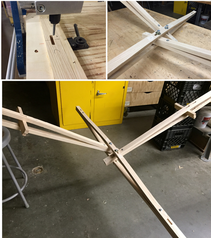
Fig. 5.9: A prototype joint, designed to test the limits of the material as required by the assembly system.
