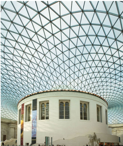
Fig. 1.3: The free-form of Foster+Partners' roof for the British Museum is developed as a response to existing edges
