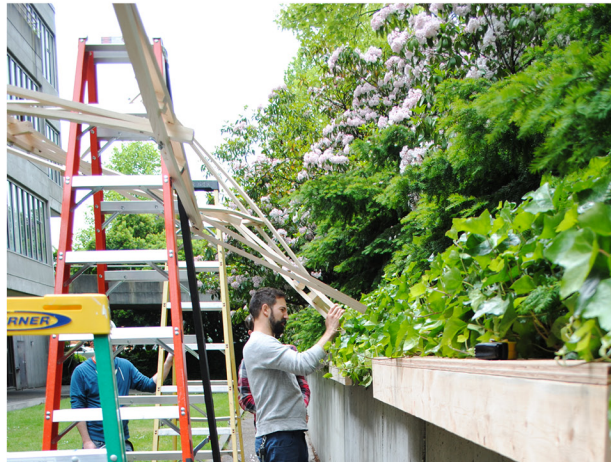
bridging to wall plates
