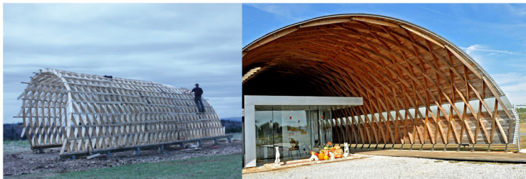
Fig 3.6: Dalhousie Coastal Studio (left) and Rural Studio (right) lamella vaults
