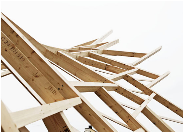
Fig 3.12: CNC fabricated full-scale prototype by Tamke et al. (2010) show the promise of axially joined assemblies.
