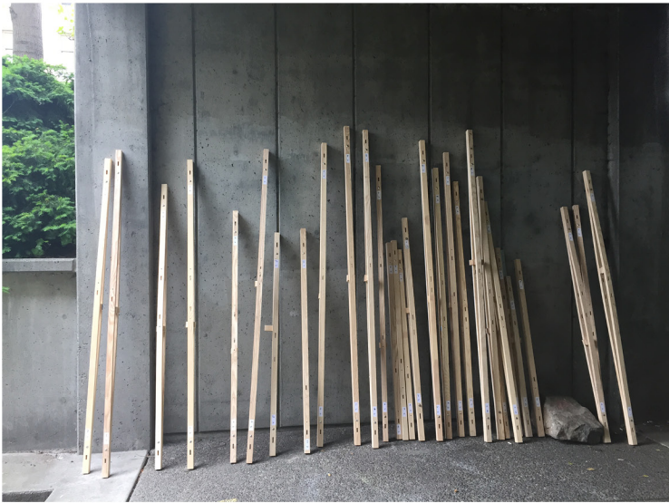
Fig. 5.20: Beams arranged in order of assembly
