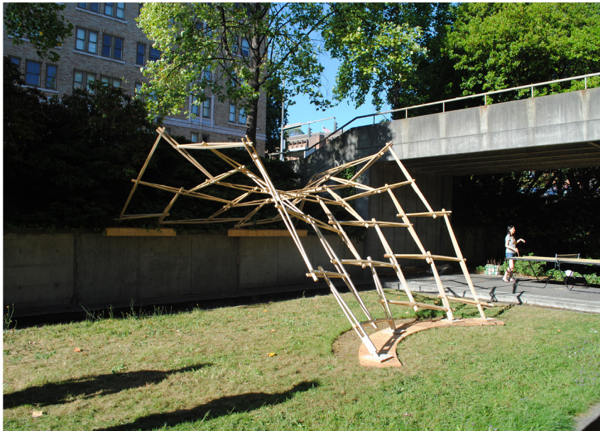
Fig. 5.26: Disassembly provided further insight into the structural requirements of the assembly. Releasing the south footing plate from the lawn, the structure did not appear to be placing significant compression or uplift on the footing. The plate could be moved, but the structure resisted this action. After releasing the north plates from the wall, the entire structure was lifted from its footings and placed on the lawn. As the scale model had done, the frame maintained its form to a great degree. Rotational resistance provided by the interleaved joints prevented the grid from twisting significantly as the model had done. When the outer edge members were removed, the grid was able to lie almost completely flat. This suggests that compression in the border of the frame was largely responsible for its form.
