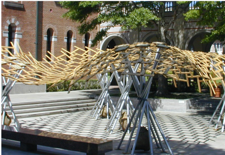
Fig 3.3: Supports of prototype structure built at Rice University
