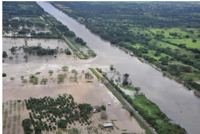
Figure 1.1. Rupture of the Dike in 2010
