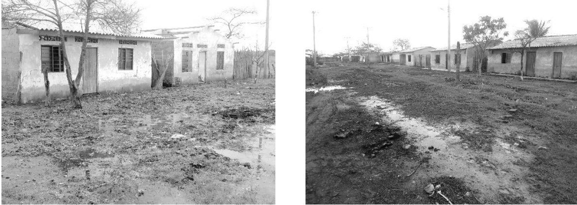
Figure 3.1. Houses Damaged by the Flood
