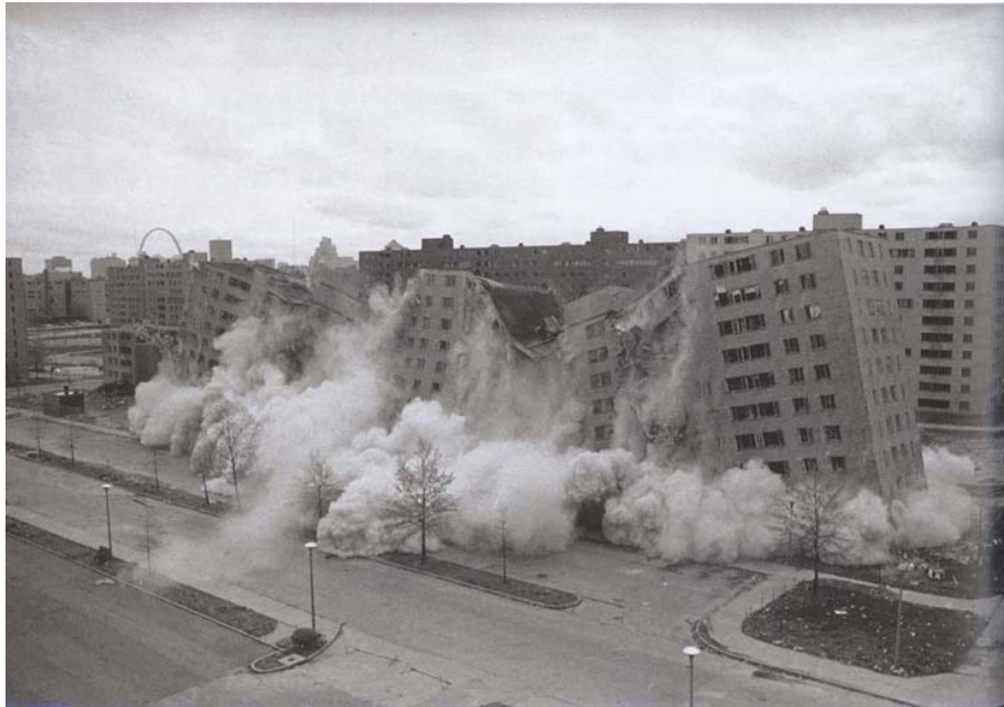
Image 5: The Pruitt-Igoe public housing project in St. Louis being demolished, April 21, 1972. Today, it is a wooded 33-acre site. 136
