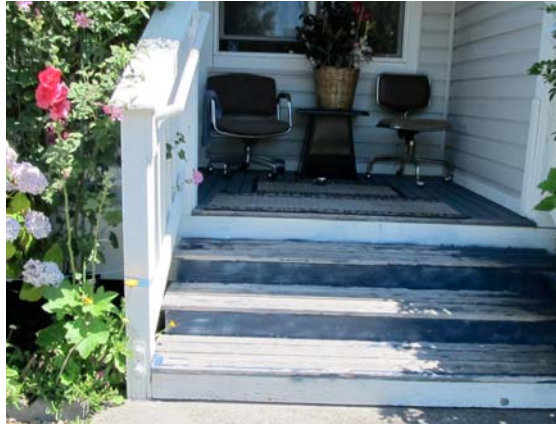
Image 22: First Two SHA-Rental Units' Porch and Stair Material Wearing and Deteriorating Compared to a Market-Rate Unit's Porch and Stair Materials with Better Quality (Third Photograph)
