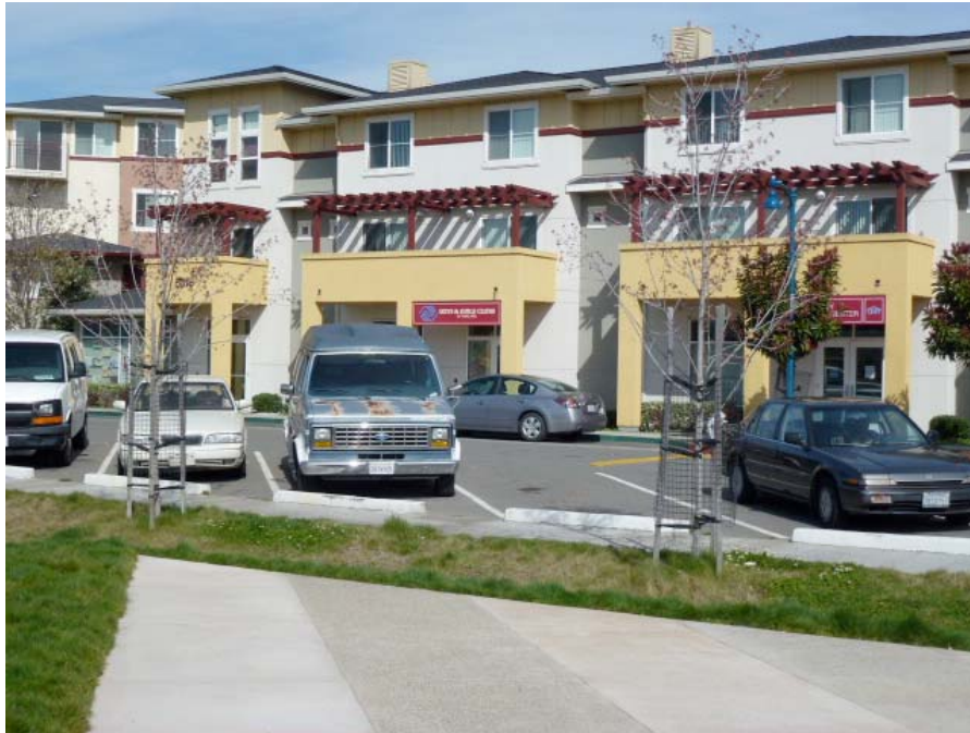
Image 34: Social Services and Child Care Building (Phase Ia), Across the Parking Lot from the Central Park
