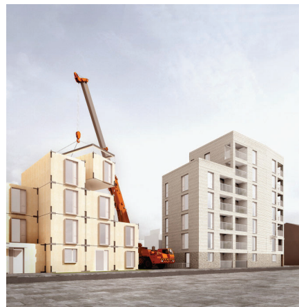
Figure 3.12: Watts Grove (2019 [construction] London, Waugh Thistleton Architects)
