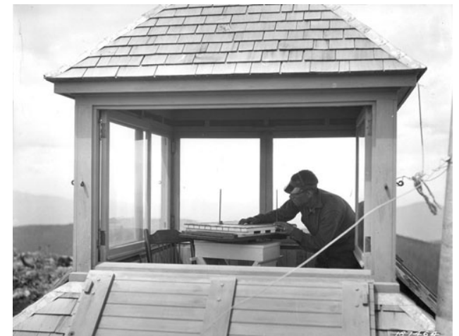
Figure 8, top: The original Mount Hood lookout, as built by Lige Coalman. Figure 9, bottom: The cupola lookout space, with Osborne Firefinder and down-swinging shutters.
