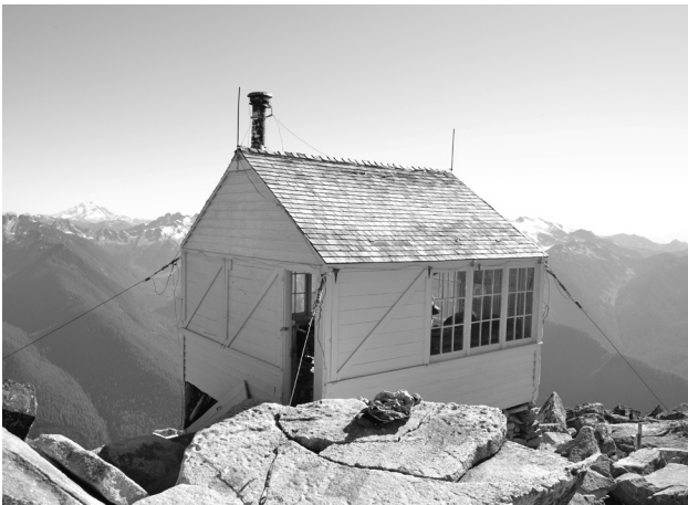
Figure 10: Hidden Lake Lookout in the North Cascades, an early gable-roofed L-4 model, built in 1931.
