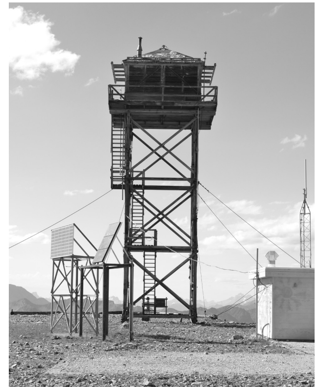
Figure 11: Desolation Peak Lookout, the earlier hipped gable L-4 model, built in 1932. Figure 12: Slate Peak Lookout, the later hipped gable L-4 with extended rafters, built in 1956.
