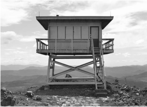
Figure 13: Red Mountain Lookout in the southern Washington Cascades, a late flat-roofed R-6 model on a short tower built in 1959.
