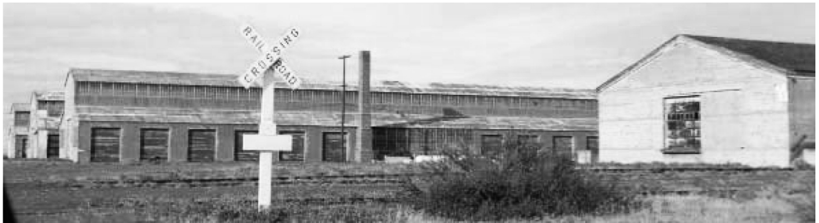
figure 9: defunct train switch yard (top of page)
