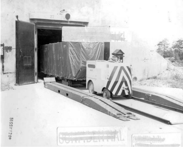
figure 12: stockpile inside storage igloos figure 13: forklifts transported stockpile
