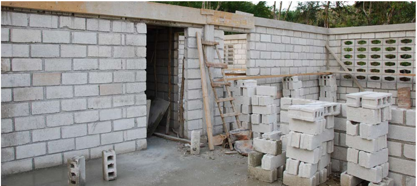
Fig. 4.6: Concrete Block Construction
