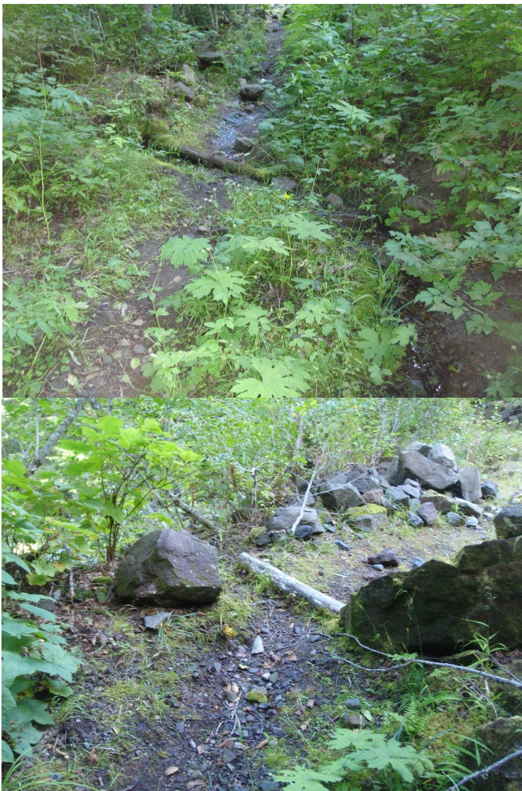
Appendix Figure 4: Point 11 and 12 Waterbars. Upper photo details the input and condition of the waterbar that I labeled as point 11. Lower photo shows the same for point 12. Note how point 12 is dry but still has scour sourced from point 11.
