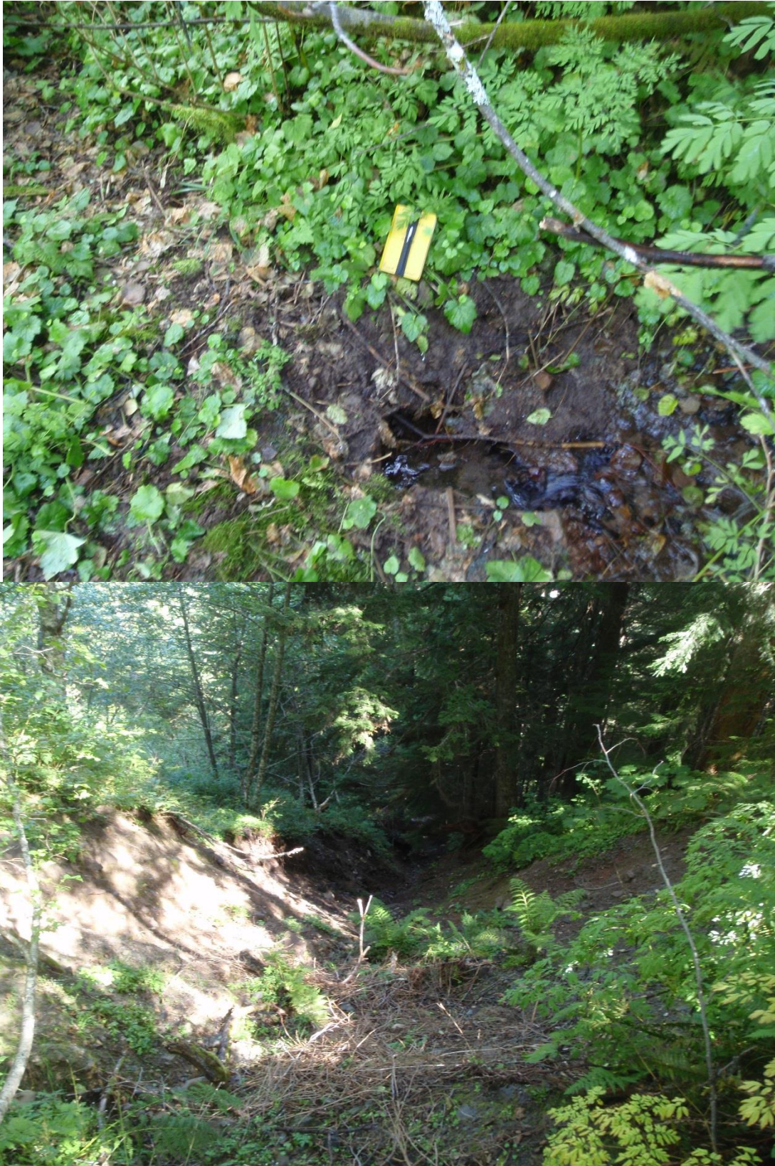
Appendix Figure 2: Photos of Point 9 Concerns. Upper photo shows the entrance to the point 9 culvert that has no exit. Lower shows the point 9 colluvial hollow emanating from the fill slope.
