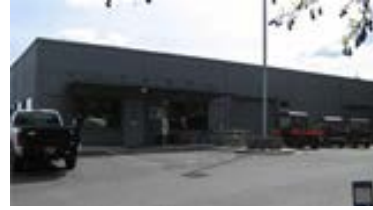
Physical Plant Building
