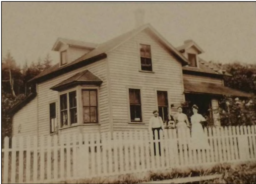
Above, an undated historic view of the Chase Residence (image courtesy of Bothell Historical Museum, "Bothell Then and Now").
