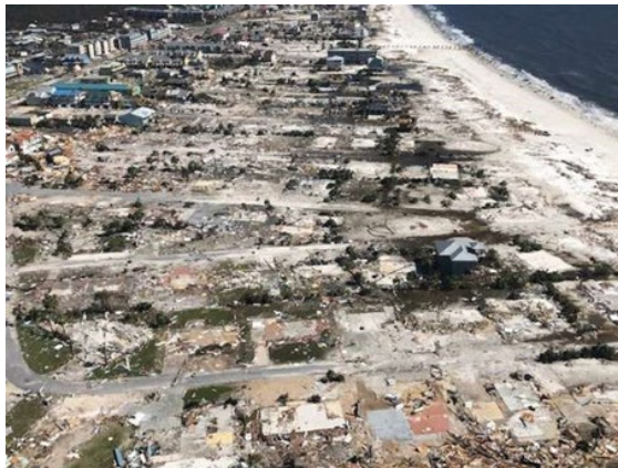
Figure 1 Image of Mexico Beach, FL after Hurricane Michael. Source: https://www.msn.com/en-us/news/world/in-florida-beach-hamlet-not-much-left-after-hurricane-michael/ar-BBOh0vo
