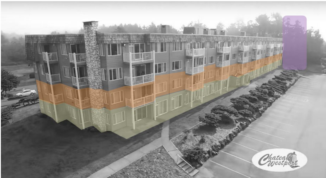
Figure 40 View of the Chateau Westport. The yellow zone indicates complete opening up of the level for flood resilience and orange zone indicates the levels that would need breakaway wall systems.
