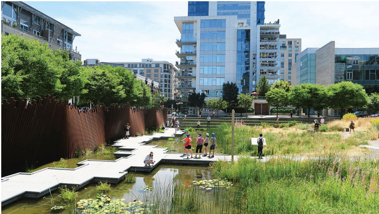
Figure 20. An example of floodable public recreational space (stormwater detention)
