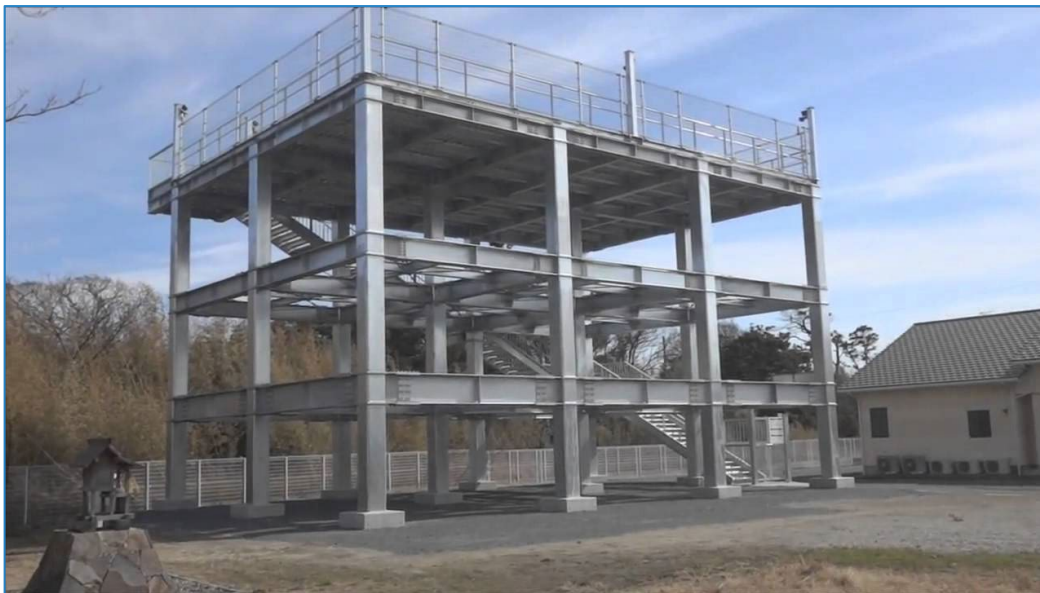
Figure 42 Example of a basic stand-alone tsunami vertical evacuation structure in Japan. Source: https://www.youtube.com/watch?v=wDh_kiVjmw4 . June 29, 2019.
