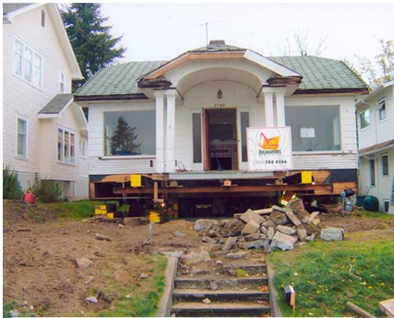
Figure 56 Phase I - A home being raised for flood prevention in Snohomish County, WA
