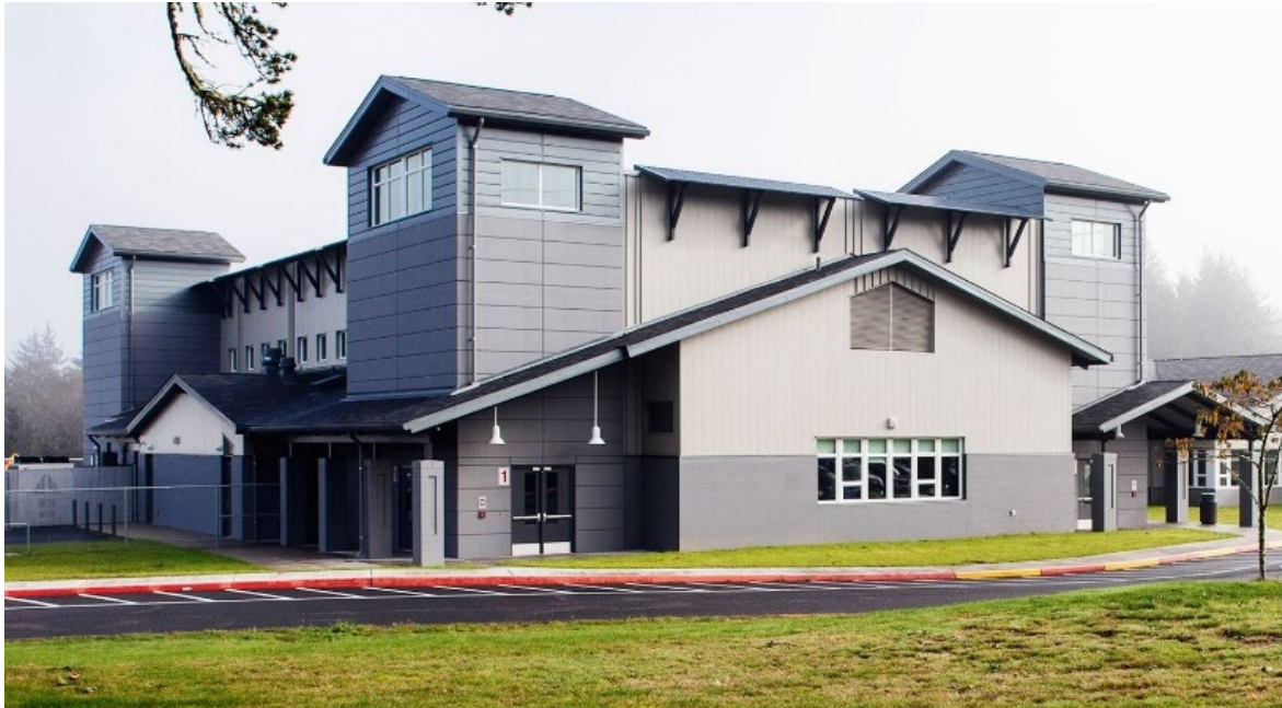
Figure 4 Ocosta School gymnasium - Nation's first structure to be designed to function as a vertical evacuation site. Source: Structure Magazine. https://www.structuremag.org/?p=14009
