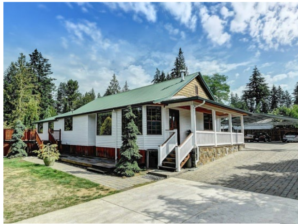
Figure 57 A home raised for flood prevention, Snohomish County, WA. Source: Zillow.com
