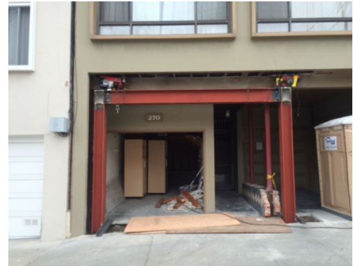
Figure 41 Examples of Soft-storey retrofits. Source: https://web.archive.org/web/20190628152803/http://www.wcpc-inc.com/soft-story-retrofit/ . June 28, 2019.
