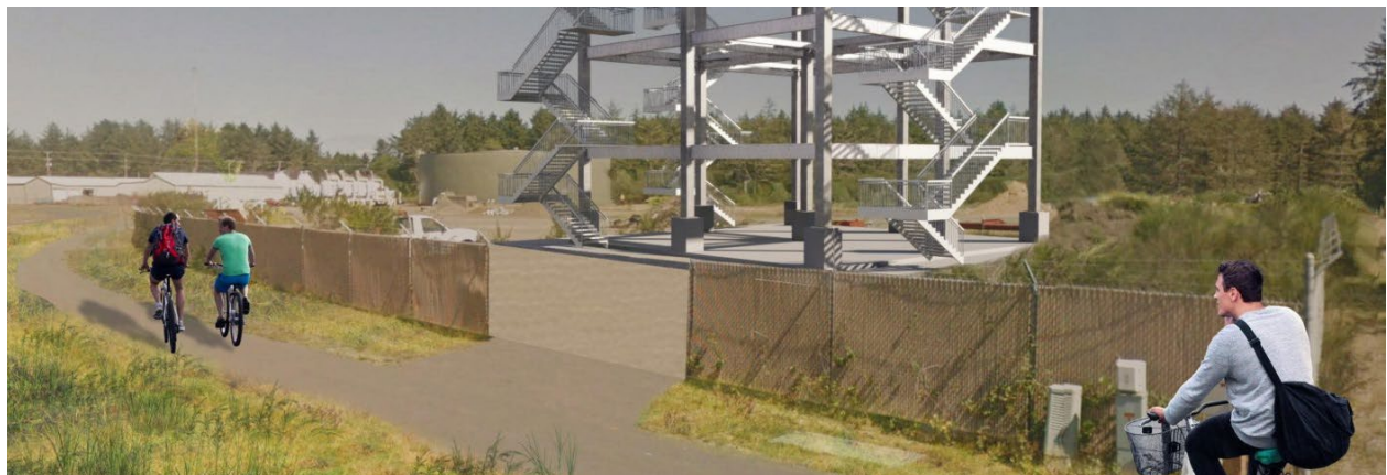
Figure 67 Conceptual design showing Vertical Evacuation structure near a biking route used everyday. Source: Degenkolb. https://degenkolb.com/projects/tokeland-tsunami-tower-conceptual-design/ . June 28, 2019.
