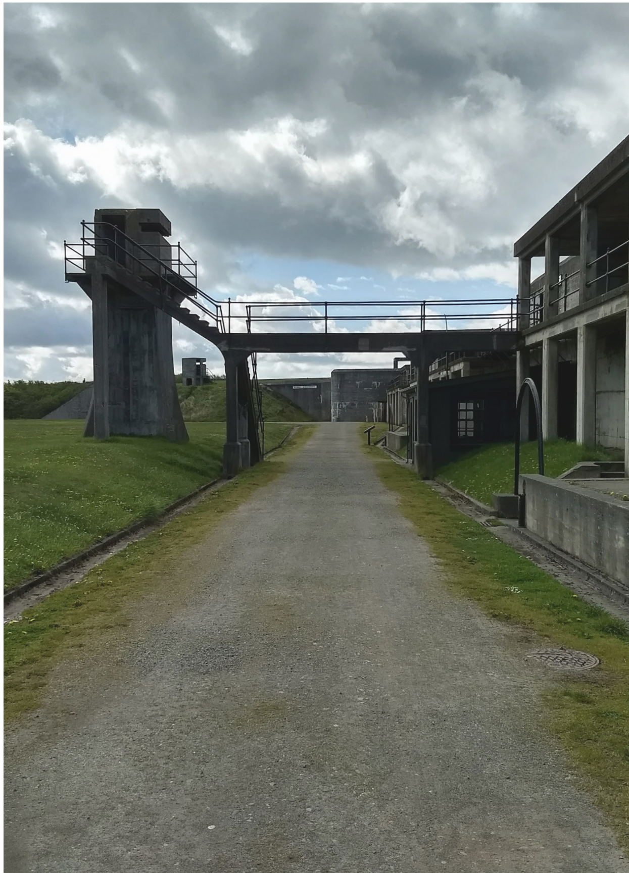
Fig. 02.1 - Batteries Worth, Moore, and Kingsbury from the access road.
