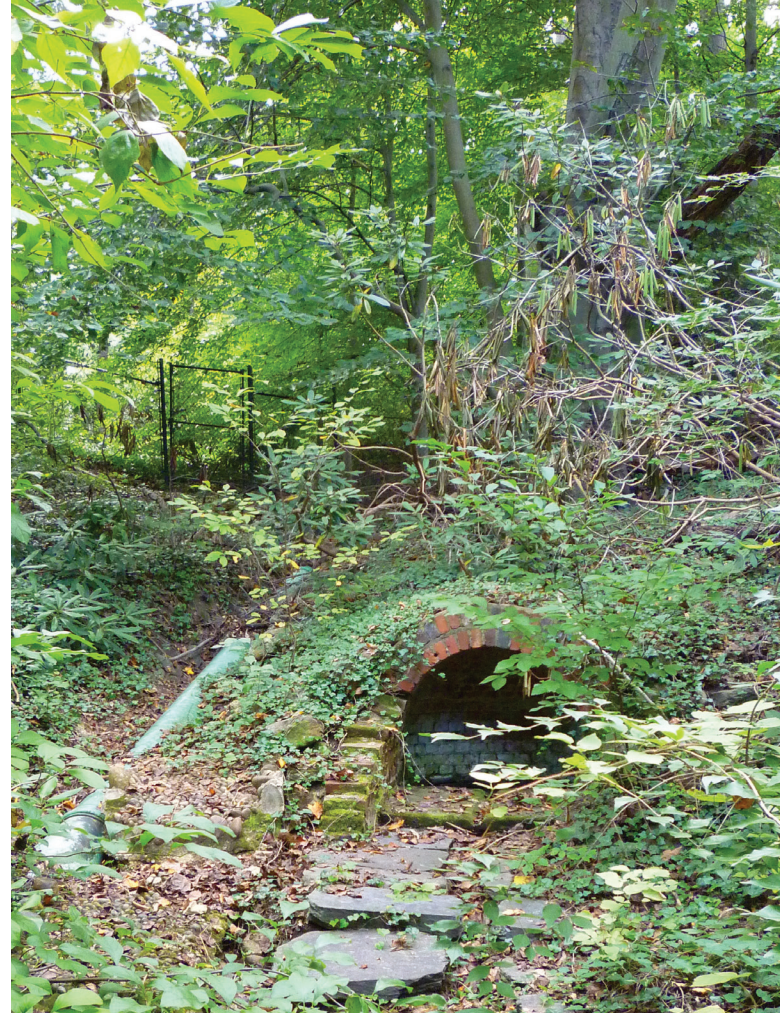
2.13 – 2.14 Farrand's design of the Pebble Stream and Stream Grotto is a functional aesthetic representation of the dual hydrologies at play in the valley. The photo on the left dates from the Bliss era and the photo above, taken in 2013, shows the degradation of the feature today. Historic photo: Dumbarton Oaks Rare Book Collection.
