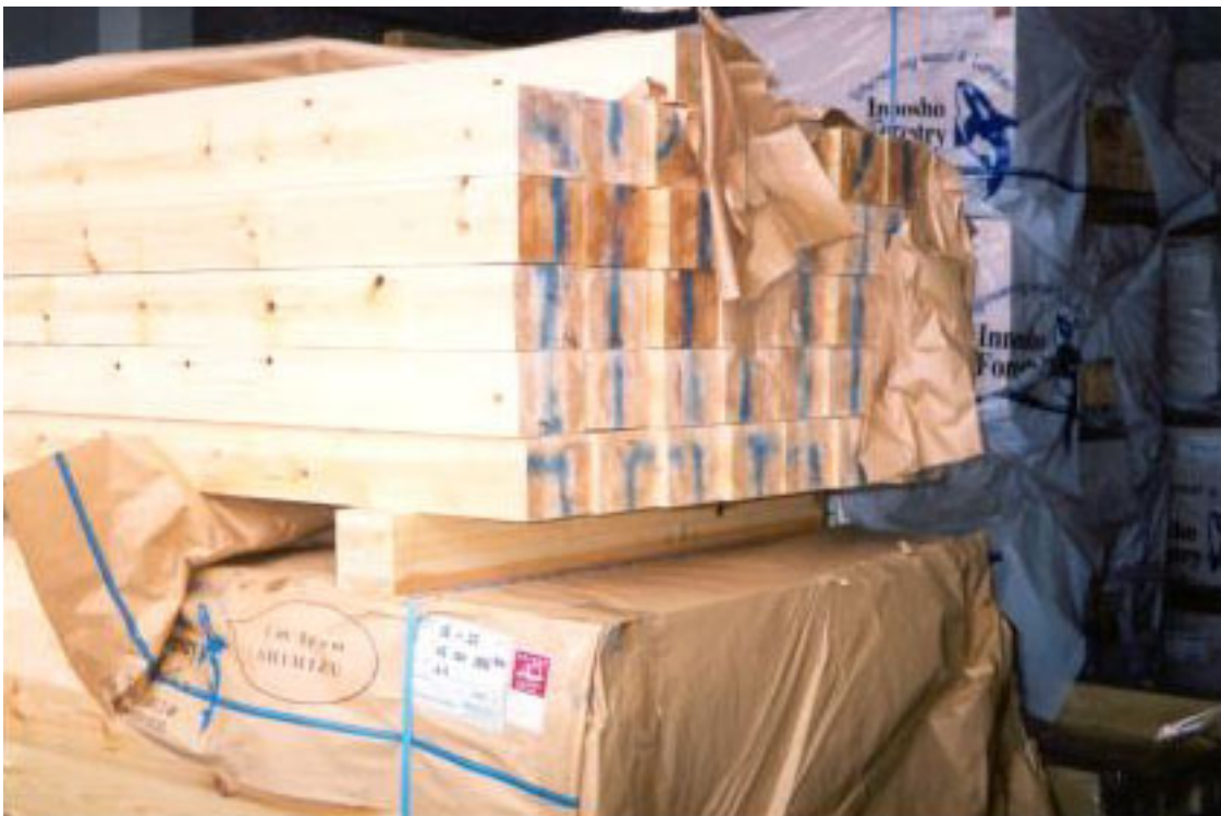
Photo 7.2. European redwood glue-laminated lumber is now treated and used for ground sills.
