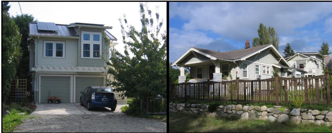
View of cottage from Phinney Ave N, looking east
