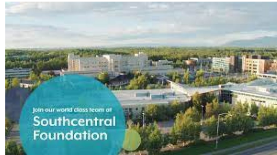
Image 12 – Aerial image of the Southcentral Foundation health campus in Anchorage, AK
