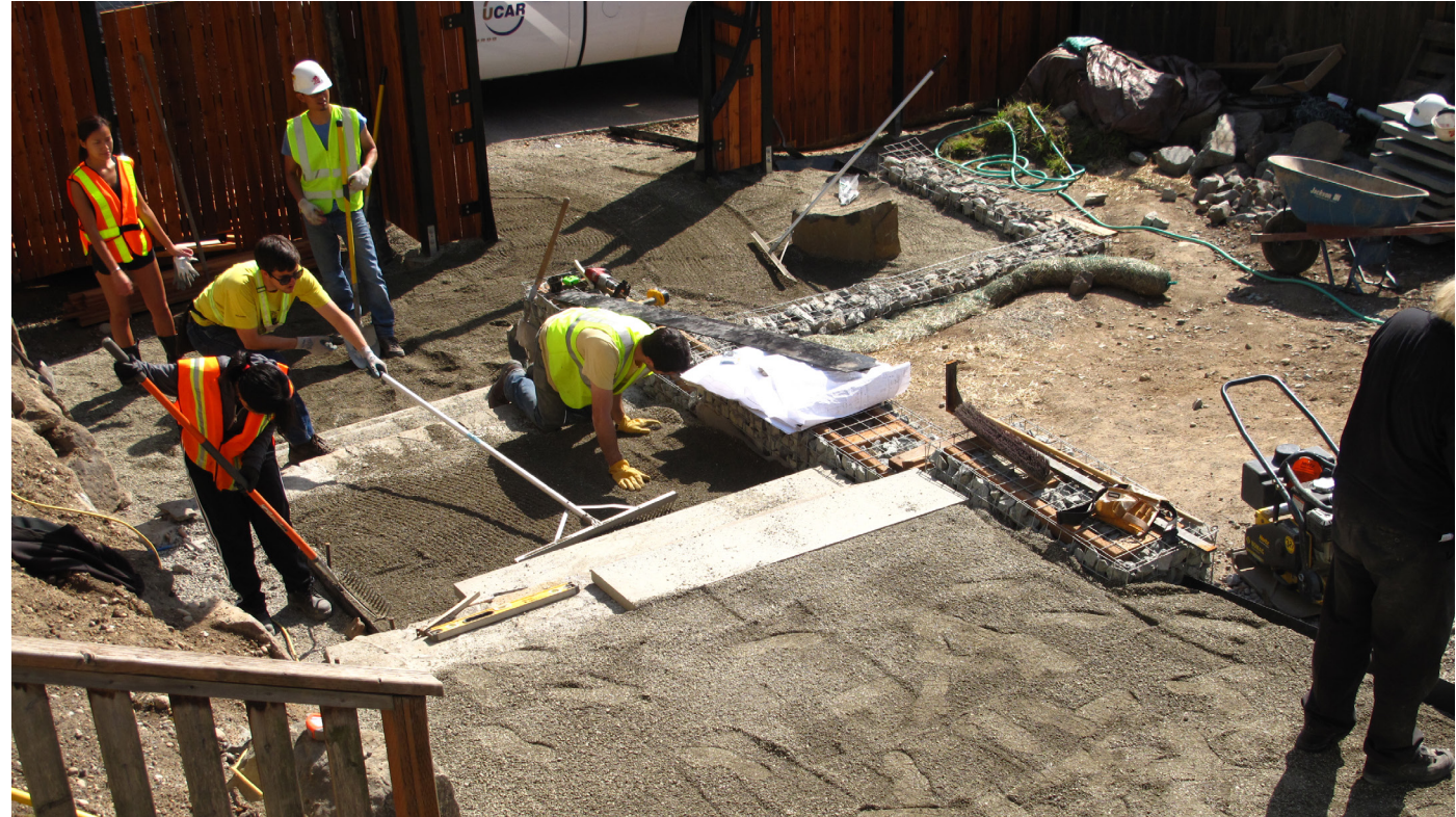
Finish grading a stair landing with a landscape rake
