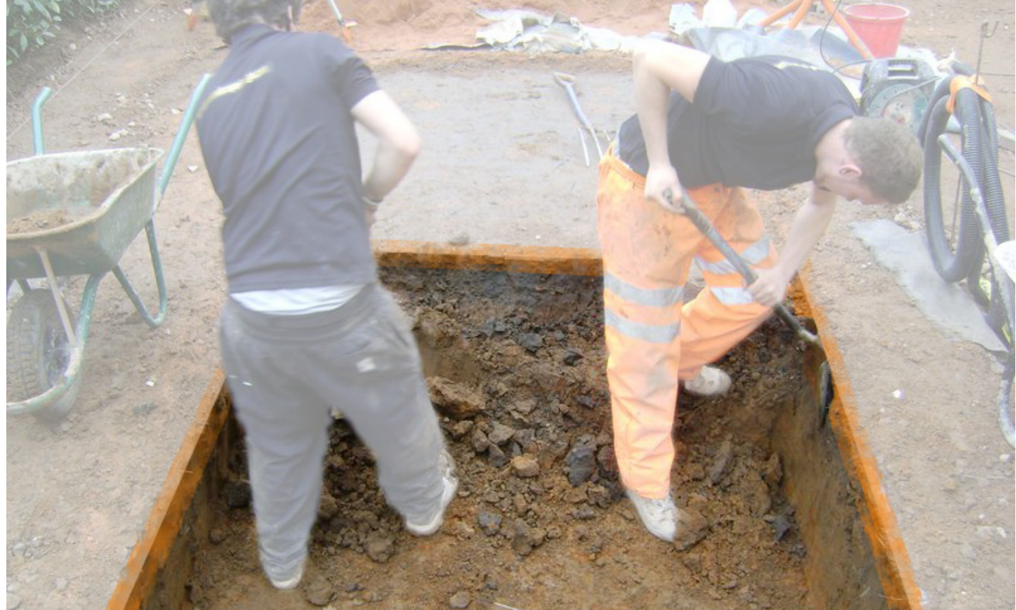
Manual excavation to establish a reflecting pond
