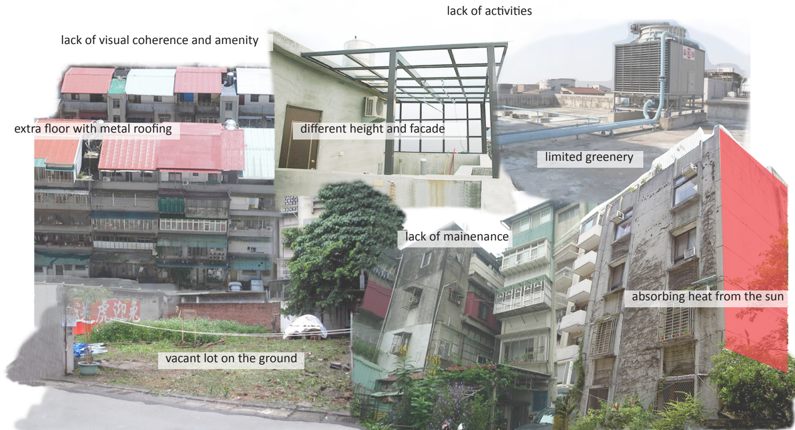
Figure 1-1: Issues related to rooftop and community open space.
