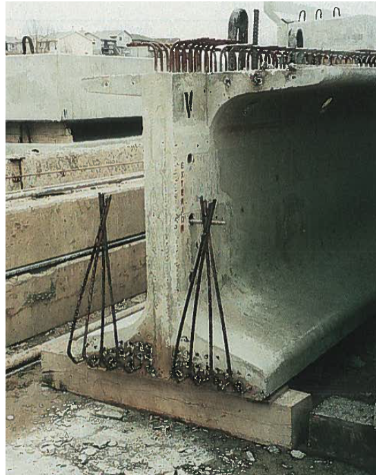
Figure 1.3: Bent Extended Strand Detail (Noppakunwijai et al., 2002)
