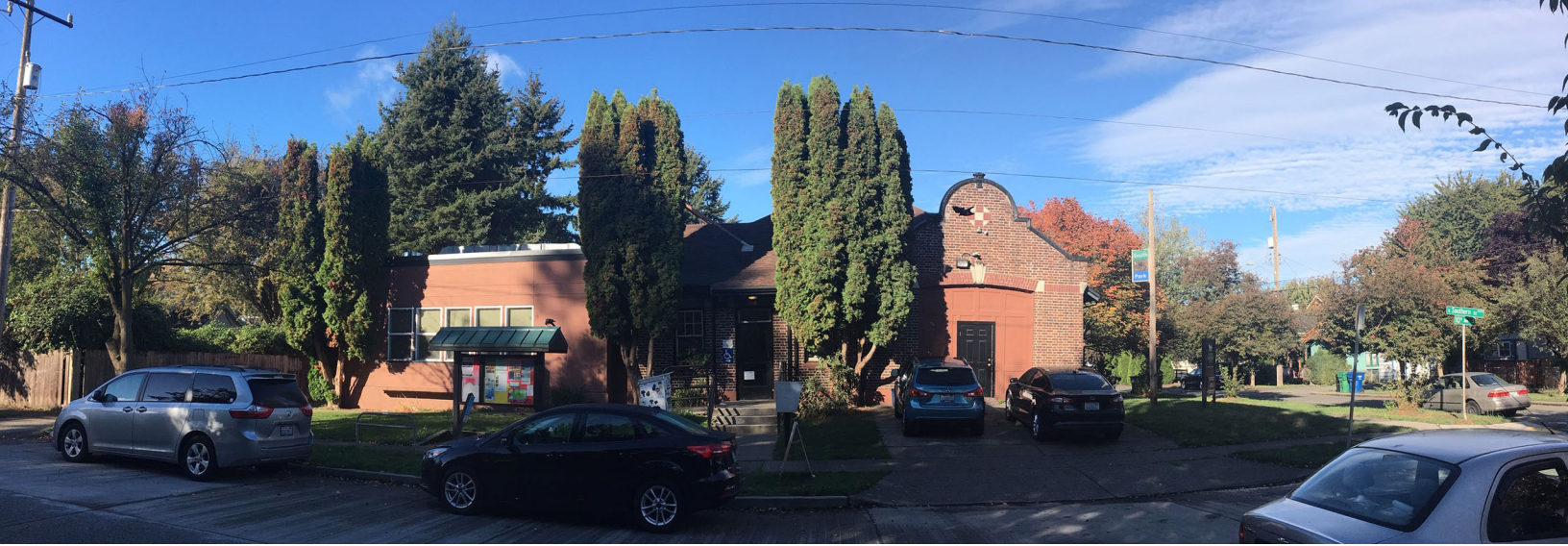
Figure 3.3 South Park Neighborhood Center panorama. Source: Stefanie Barrera Aguila.
