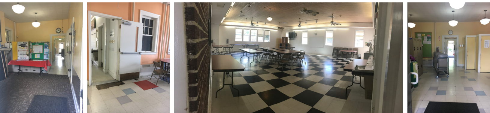
Figure 3.5 Interior condition of the South Park Neighborhood Center. The corridor is the area where children stay while their parents attend workshops. Source: Stefanie Barrera Aguila.
