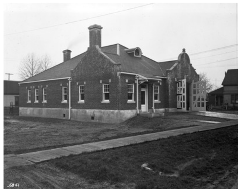
Figure 3.4 Historic image of South Park Neighborhood Center. Source: Washington State Department of Archaeology and Historic Preservation.
