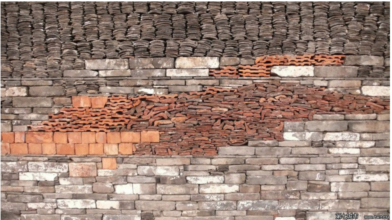
Figure 11. Traditional tile facade, designed by Wang Shu, image © Evan Chakroff
