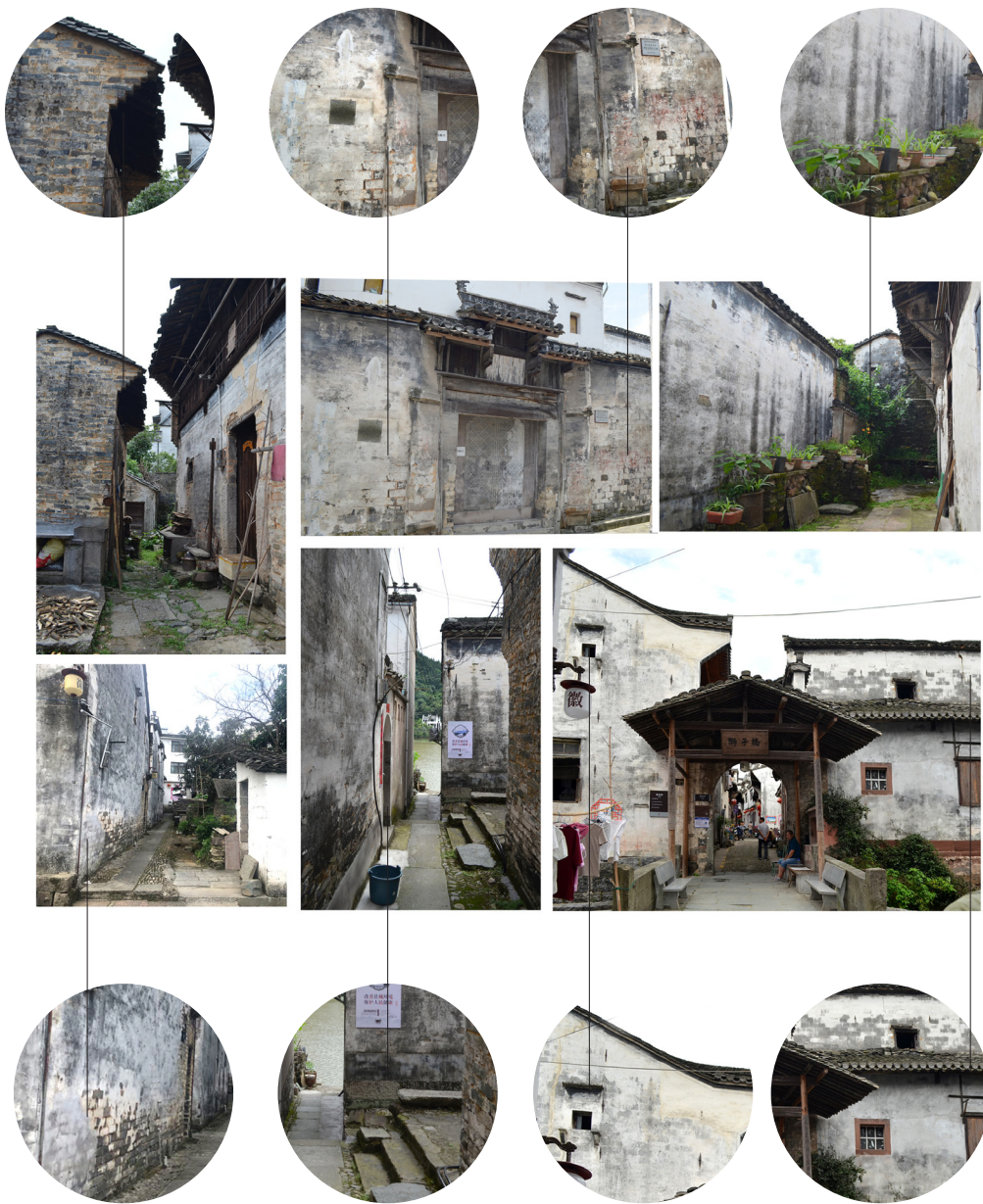
Figure 58. Existing Cladding Texture
