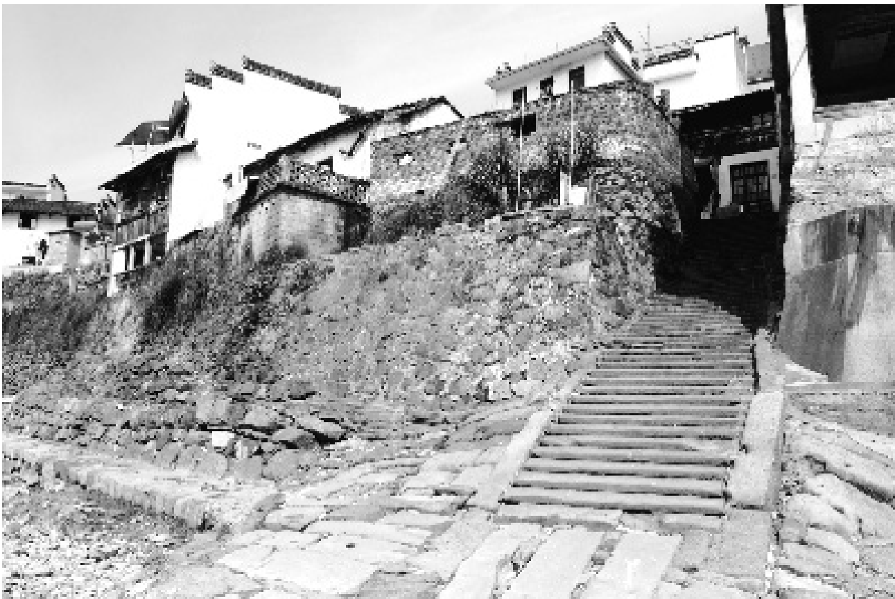
Figure 55. Stairs at Waterfront
