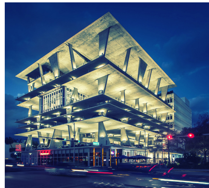
Figure 5.14 - 11 11 Lincoln Road parking garage in Miami, FL
