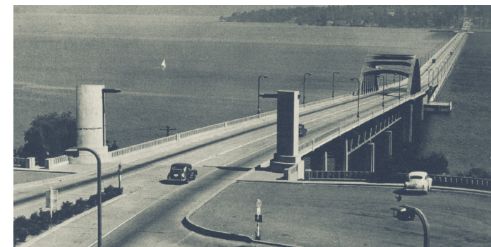
Figure 4.22 - The floating bridge forming Interstate-90 opened in 1939
