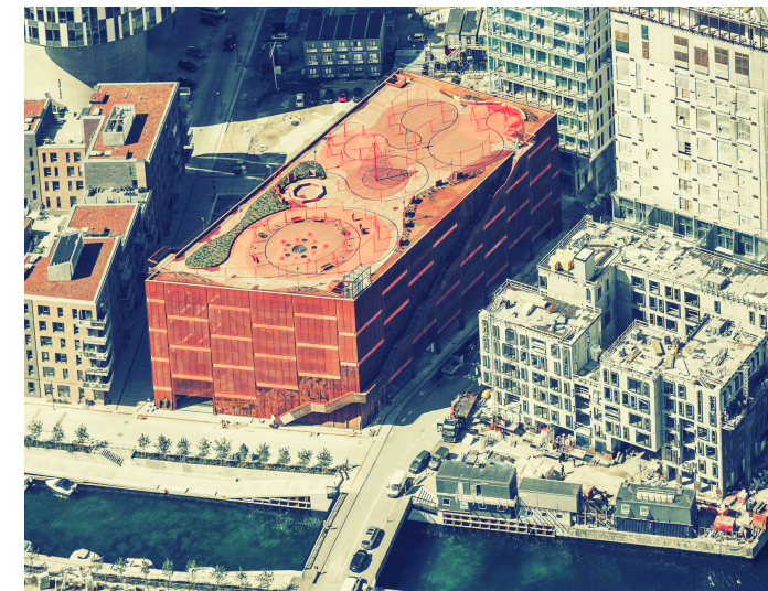
Figure 5.19 - Park 'n' Play with play area on the roof of a parking garage
