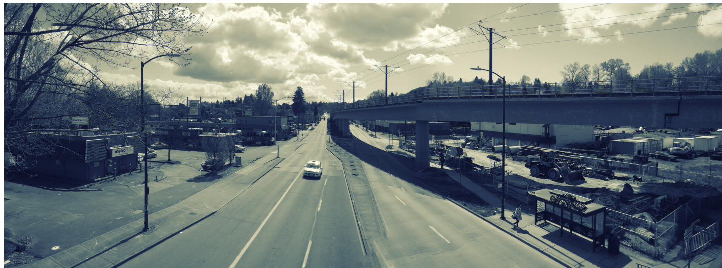
Figure 6.4 - Overlooking Martin Luther King Jr Way S running parallel with the elevated light rail tracks
