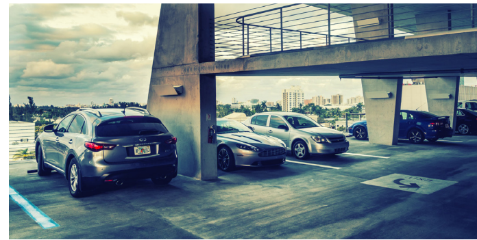
Figure 5.15 - Lincoln Road parking garage during normal business hours
