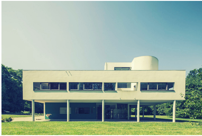
Figure 3.A.11 - Villa Savoye in Poissy, France designed by Le Corbusier
