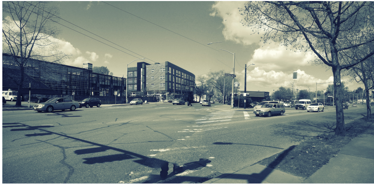
Figure 6.3 - Overlooking the Mount Baker light rail station at the intersection of Rainier Avenue S (left) and Martin Luther King Jr Way S (right)
