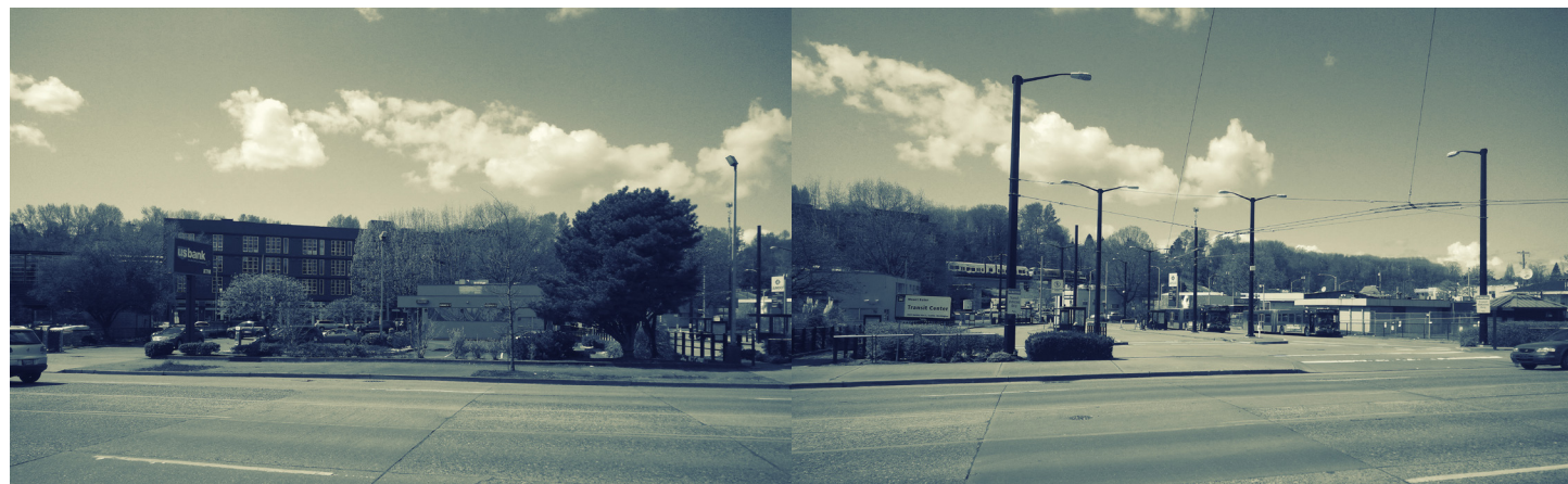
Figure 6.5 - Overlooking parking lot for Starbucks and US Bank adjacent to the bus transit center, the light rail station is in the background
