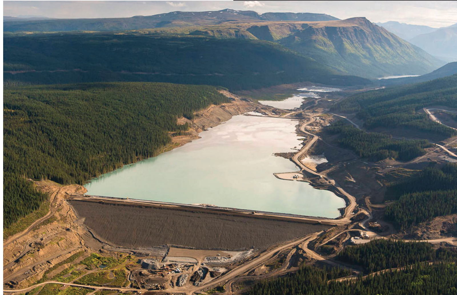
FIGURE 7- Red Chris Mine tailings storage facility and earthen dam (Source: Juneau.empire)
