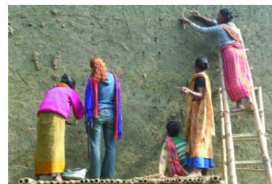
Figure 75: the 'Hand Made' construction
