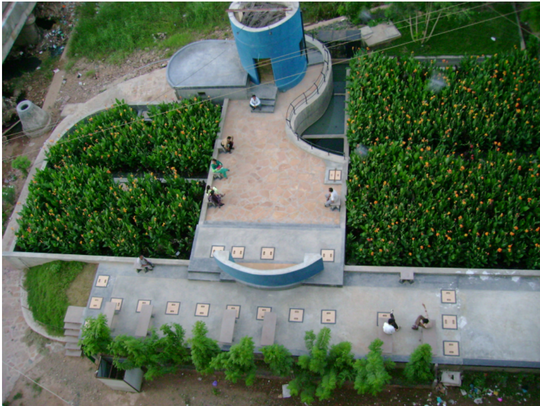
Figure 68: In Bhuj, recycled water from a decentralized wastewater treatment system is used to create a green-belt. Photo from Hunnarshala.
