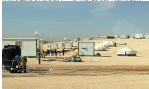
Figure 23: Zaatari camp in the new established areas in the south west of the camp. January 2014.
