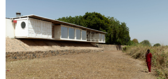
Figure 70: A series of shipping containers make up the accommodation block for staff, @ TAMassociati
