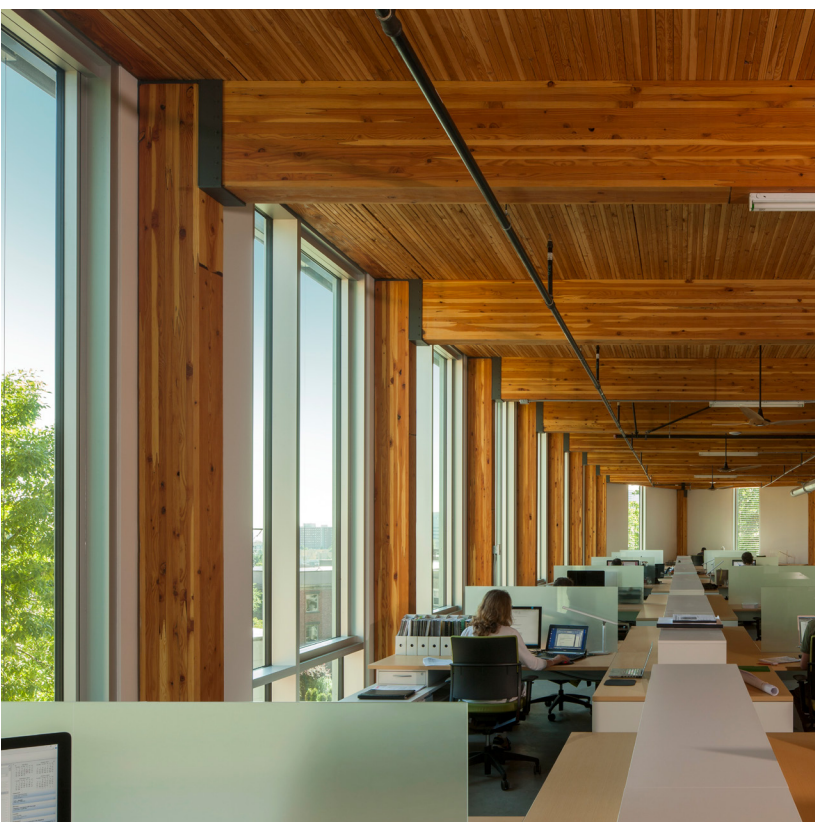
Fig 3.2 Heavy timber in the Bullitt Center co-working space
