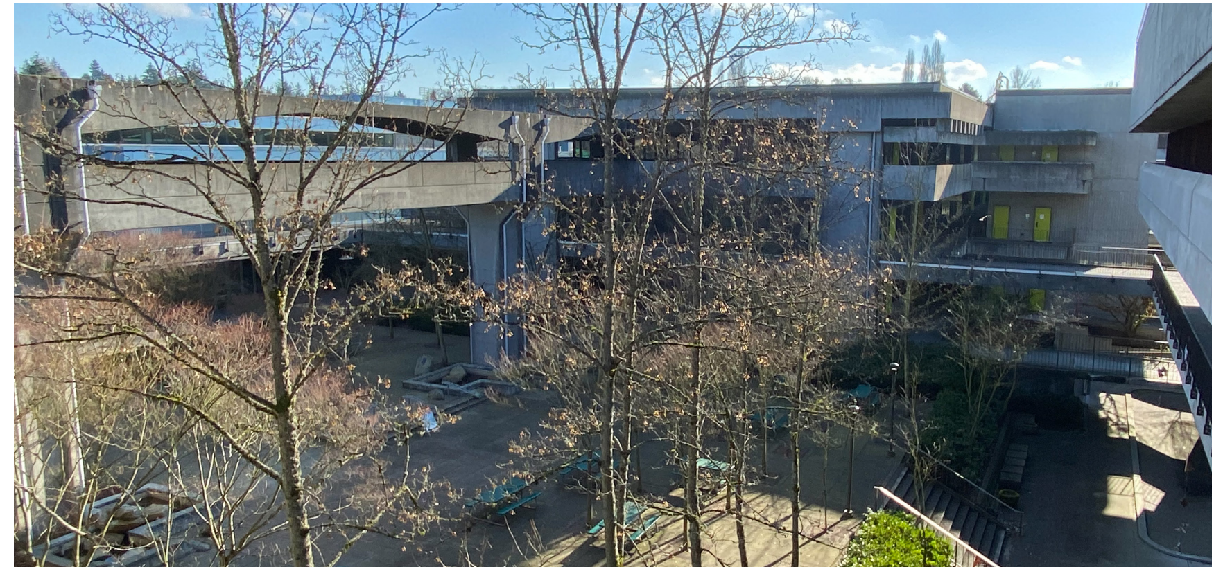
Fig 4.9 Interior courtyard at NSC looking south toward the third floor bridge
