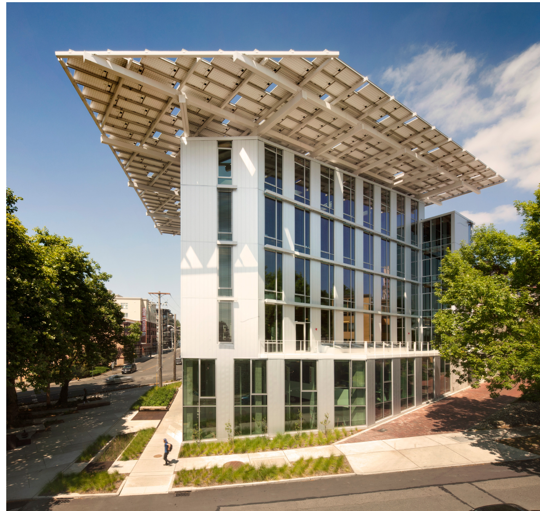
Fig 3.3 The Bullitt Center in Seattle, WA
