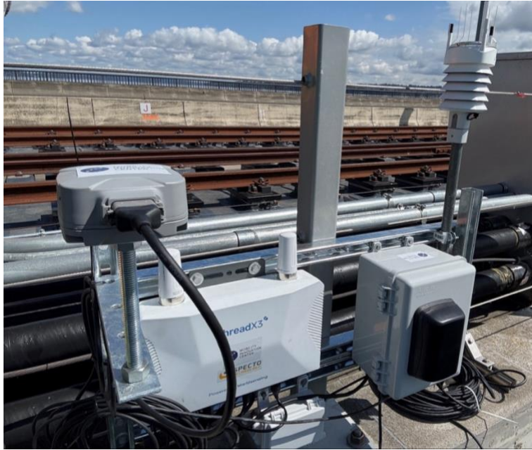
Figure 10. Long-term monitoring setup at bridge midspan (Pontoon J)
