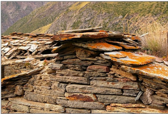
Figure 21: Slate is the traditional roofing material used in the Johar Valley.
