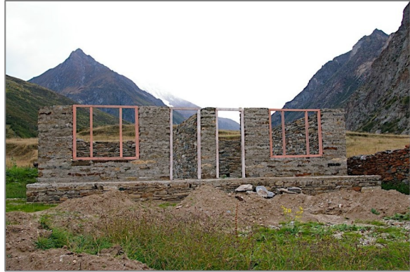
Figure 51: KMVN guesthouse under construction in Martoli.
