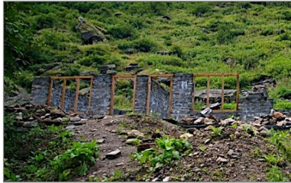
Figure 35: KMVN guesthouse under construction.
