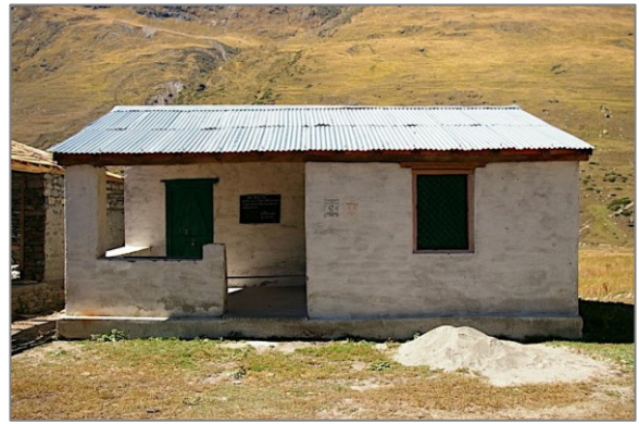
Figure 22: Some new construction in Burphu does not conform to traditional style or roofing materials.
