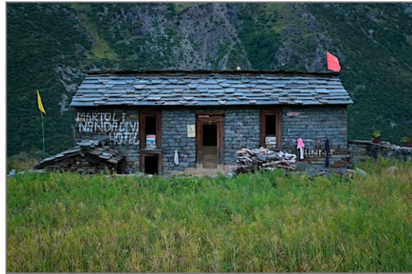
Figure 24: Guesthouse in Martoli. The upper floor is used to house visitors.
