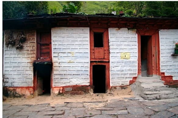
Figure 30: Traditional architecture in Lilam. Intricate woodcarvings were painted rust orange.
