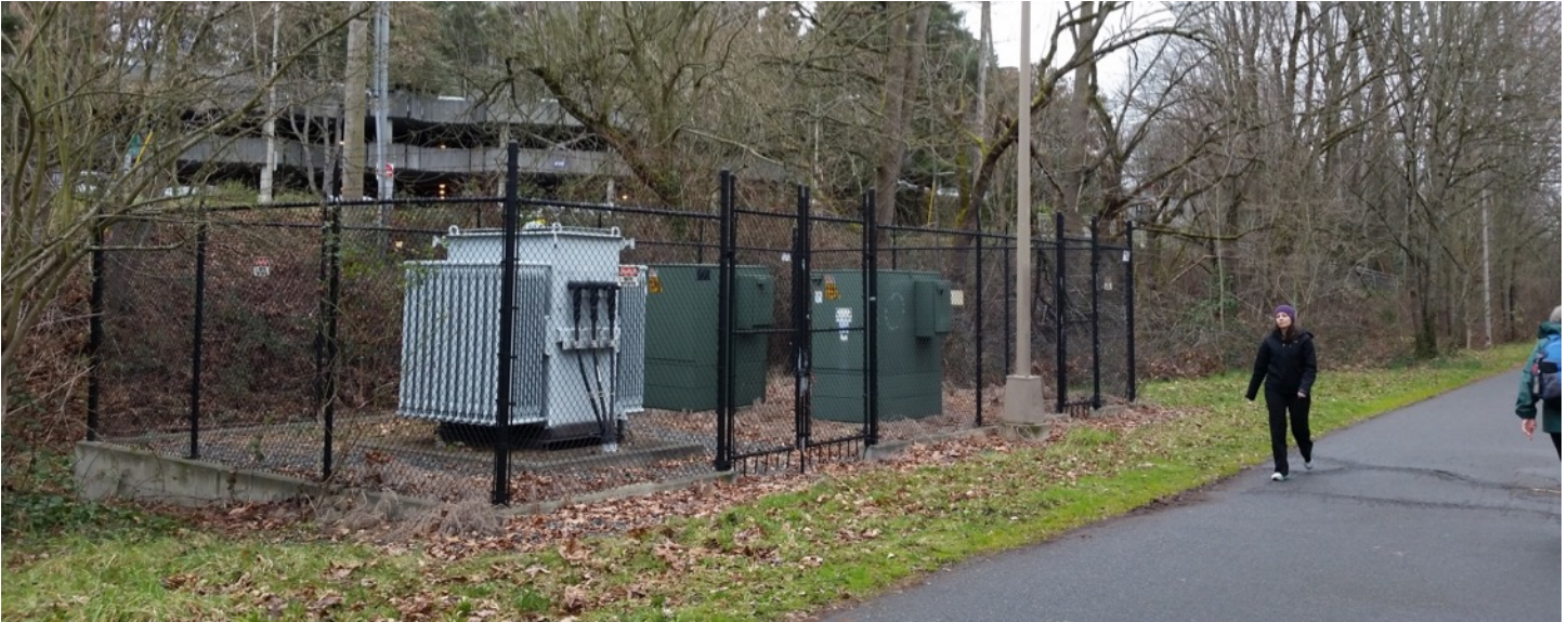
Figure 8: Fenced Off Utility Boxes
