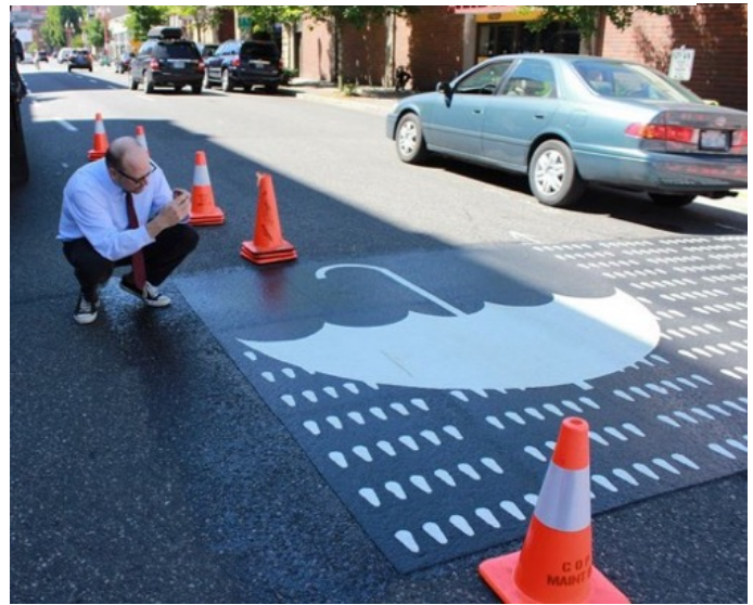
Figure 34: Portland Raindrop Crosswalk
