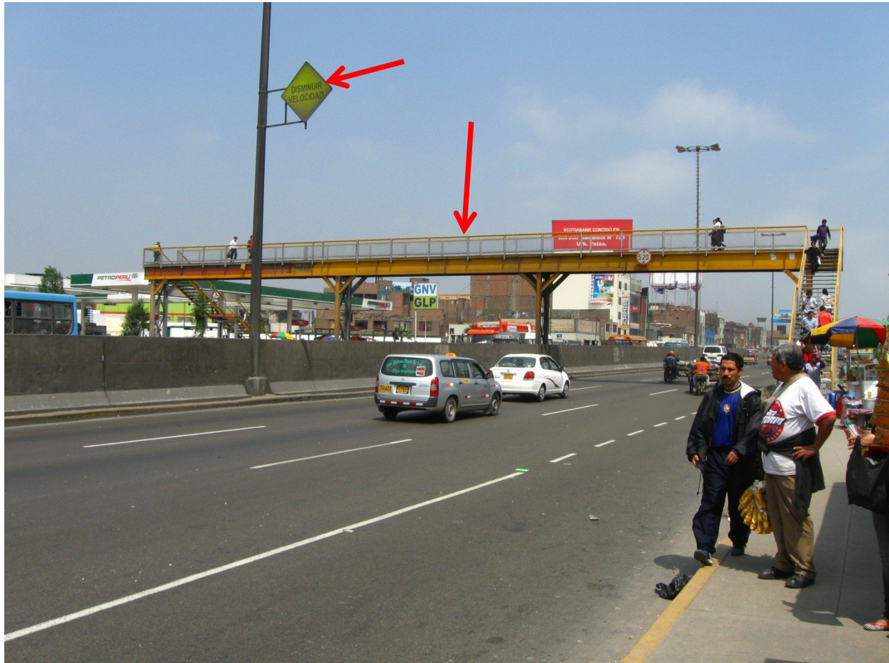
Figure 13. Example of a pedestrian bridge over the Panamerican Highway and a “Slow Down” (Disminuir Velocidad) sign.
