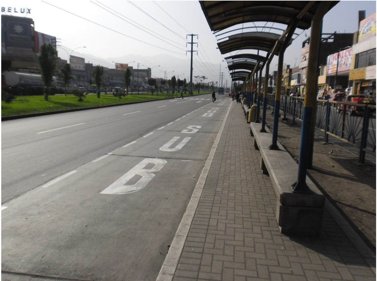
Figure 8. A bus stop with a bus bay or pullout area allowing buses to exit moving traffic to board and alight passengers.
