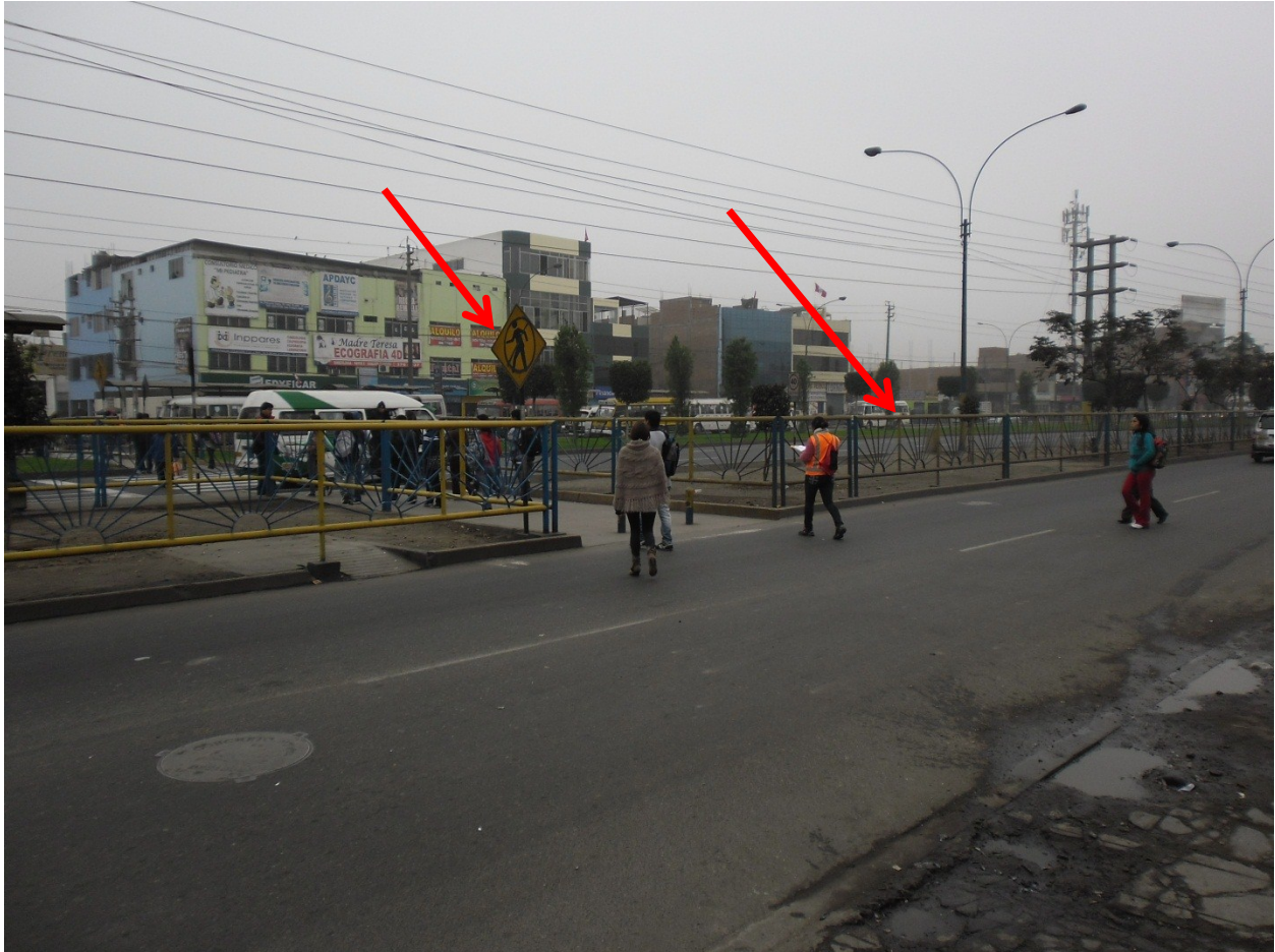
Figure 10. Mid-block crossing with pedestrian barricades and a (modified) pedestrian crossing sign.
