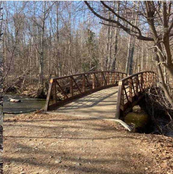
The sight when emerging from backyards, entering public park space
